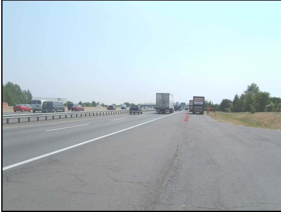
Figure 33. Photo of Extra Wide Paved Shoulder.
