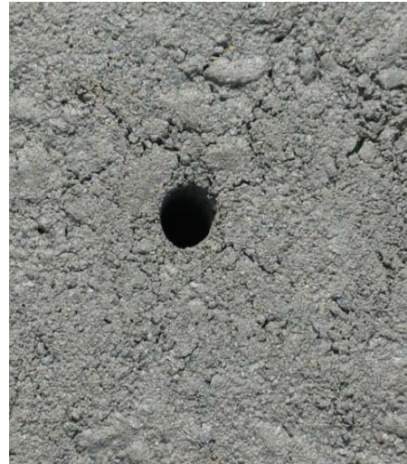
b) cracks induced before density test
