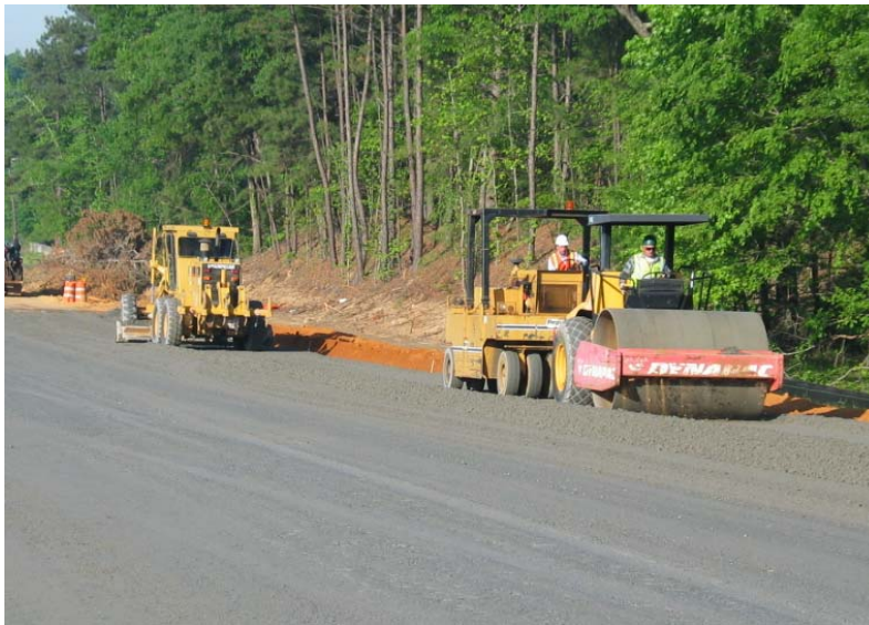
Figure 36. Compaction Sequence on SH 31.
