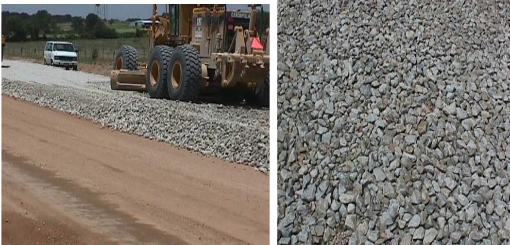
Figure 31. Construction of the Large Stone Base on FM-1810.
