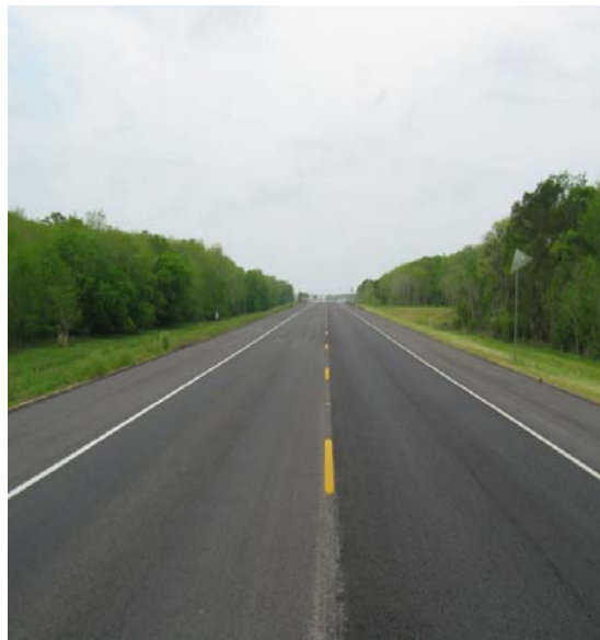
b) after placement of HMA
