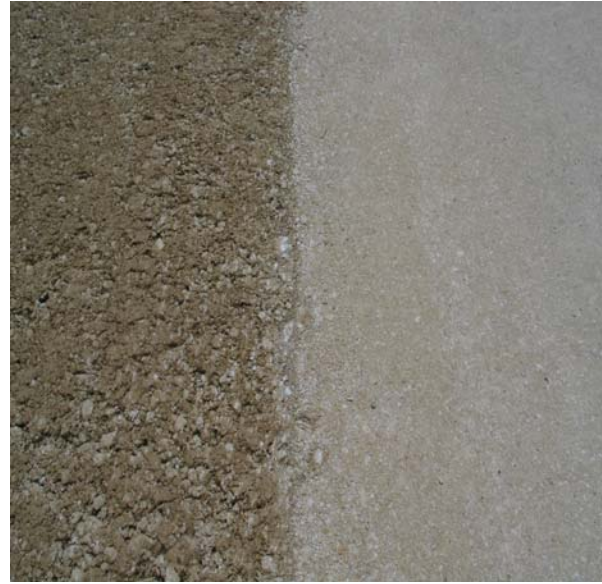
b) Joint in placed base
