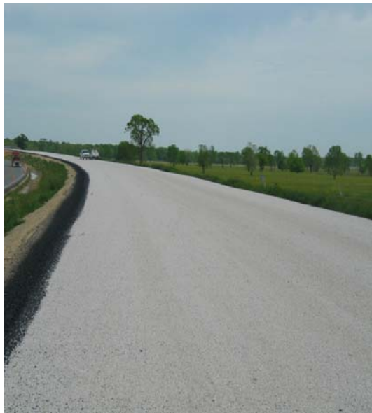
a) Underseal prior to HMA placement
