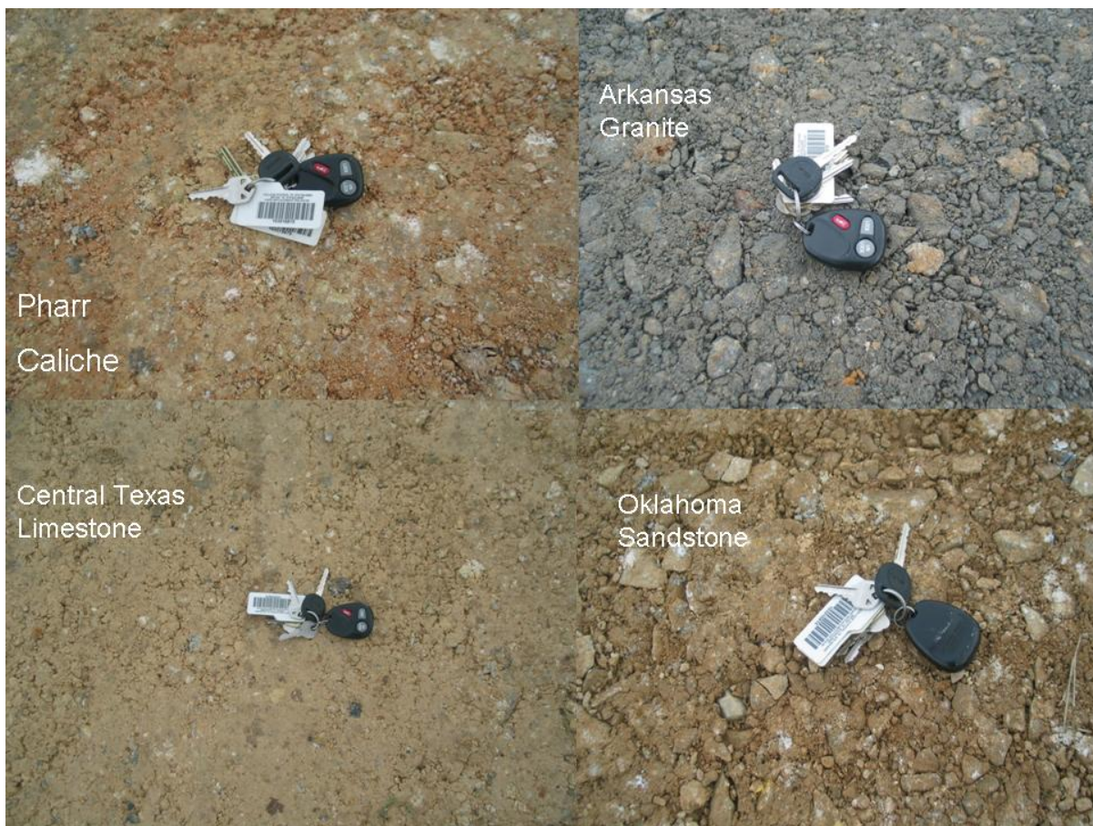
Figure 1. Visual Appearance of Existing Item 247 (left) and Item 245 Bases.
