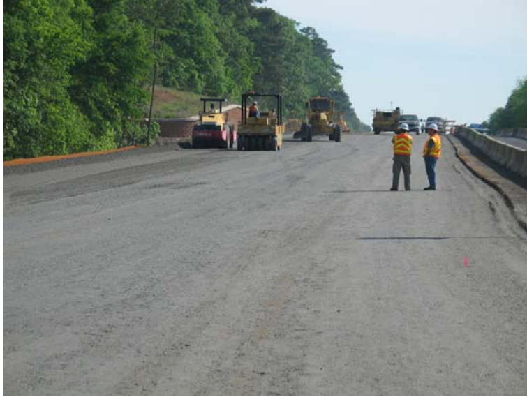
Figure 35. Arkansas Granite Base Being Placed on SH 31.
