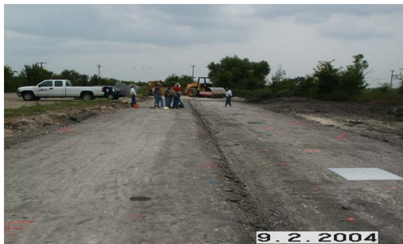
Figure 43. Subgrade Just Prior to Base Placement.
