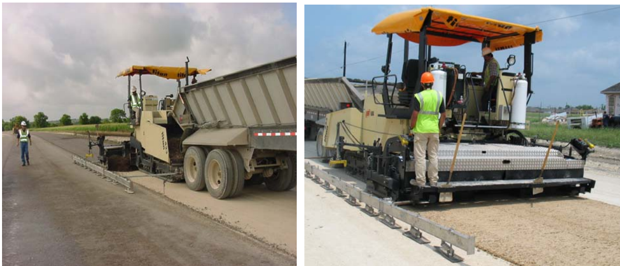
Figure 57. Base Paver Operations in the Waco District.
