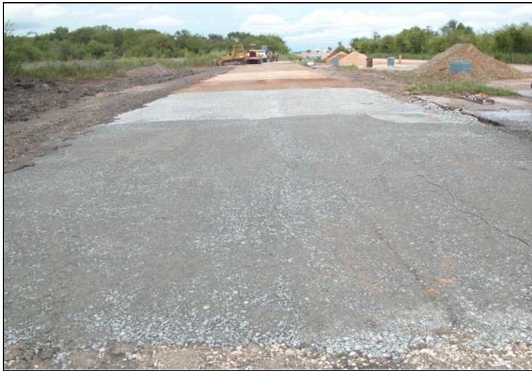
Figure 44. Completed Base Section at TTI's Riverside Campus.
