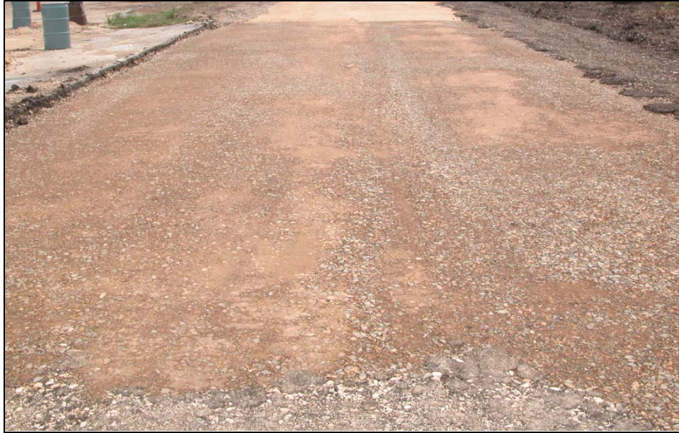
Figure 21. Test Sections Built with Sawyer Pit Material.
