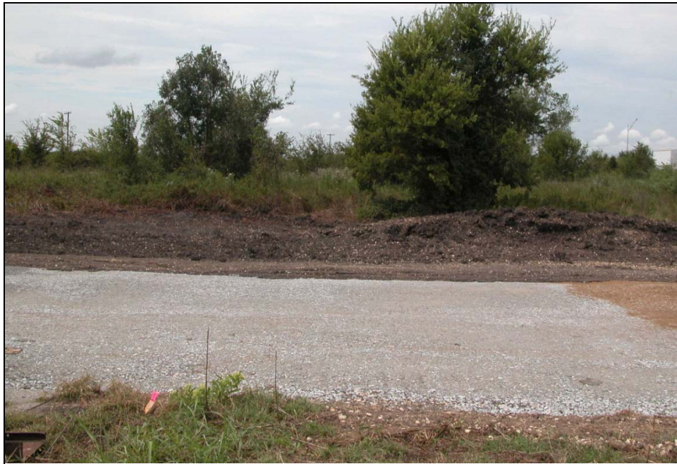
Figure 20. Test Section Built with Springdale Material.
