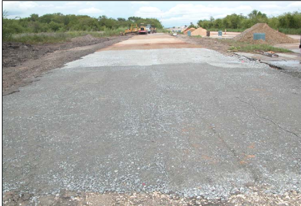
Figure 18. Test Sections Built at Texas A&M University Riverside Campus.
