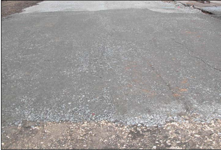
Figure 19. Test Section Built with Granite Mountain as Base Material.
