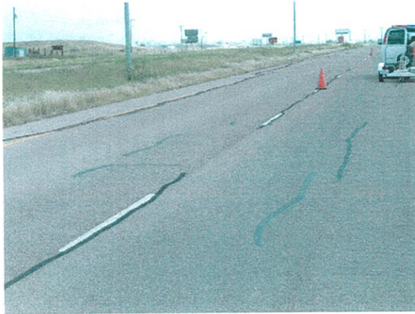
1. Typical sealed cracks in middle of lane
