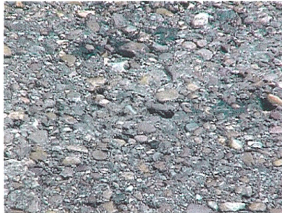
Segregation on patched area. Patch 25 X 12 feet.
