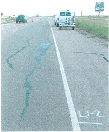
1. Patched failure
