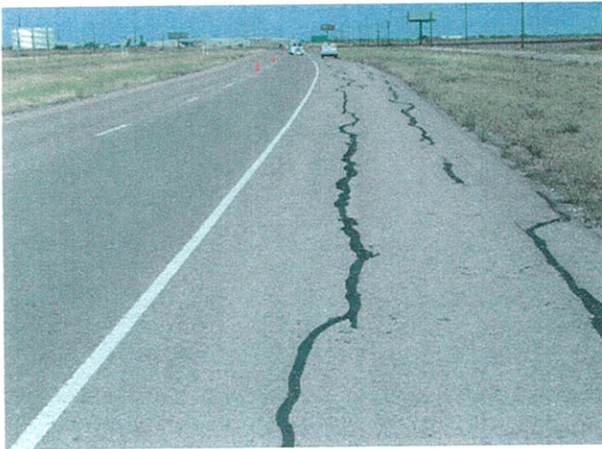
1. Sealed cracks on shoulder
