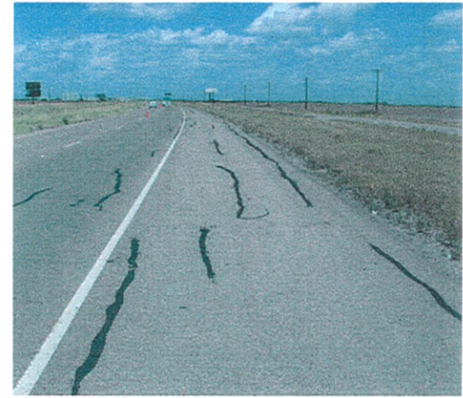
4. Sealed cracks on shoulder
