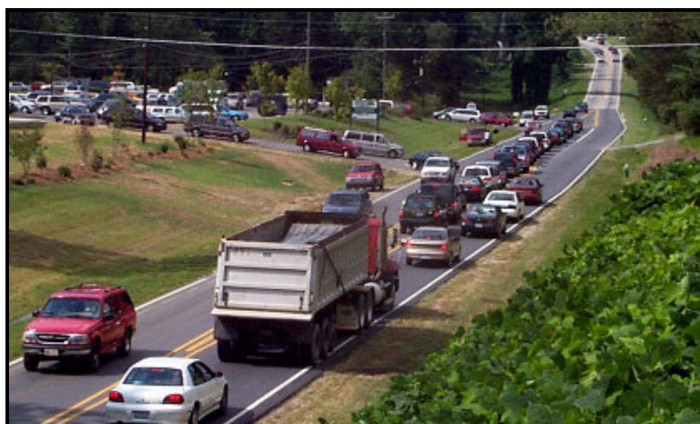
Figure 52. Queue in Left-Turn Lane Starting to Spillback and Block Through Lane.
