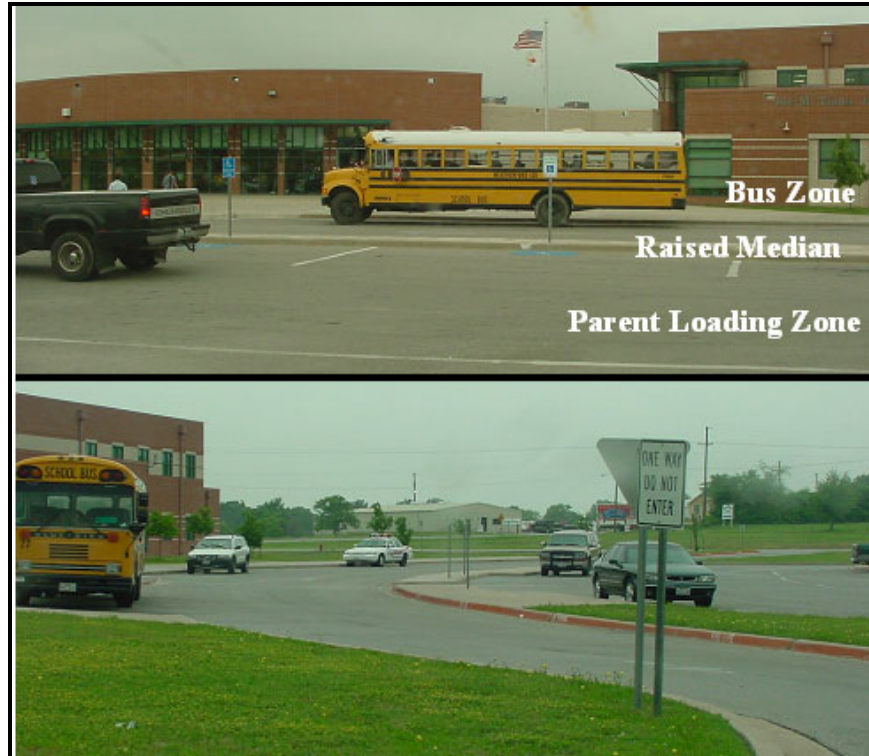
Figure 16. Site with a Layout to Avoid – Bus and Parent Zones Adjacent to Each Other.
