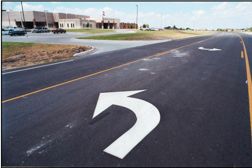
Figure 53. Newly Installed Left-Turn Lane in Front of an Elementary School.
