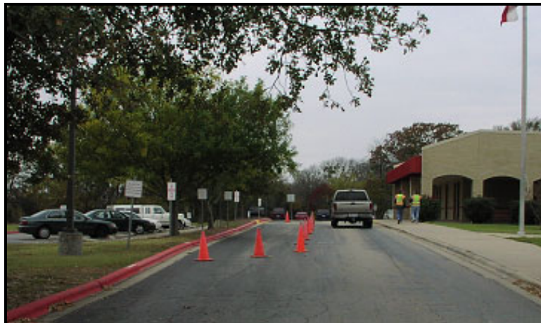
Figure 33. Placement of Traffic Cones to Create a Single-Lane Queue.
