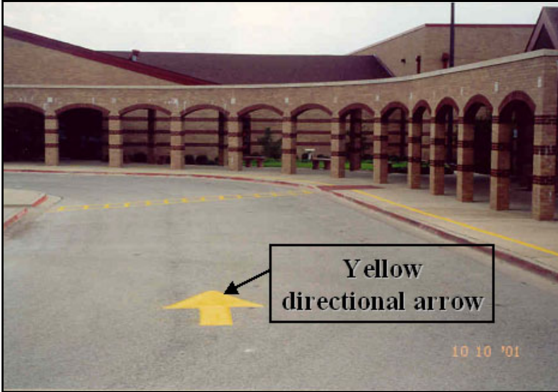
Figure 54. Example of Yellow Markings for On-Site Crosswalk at Elementary School.
