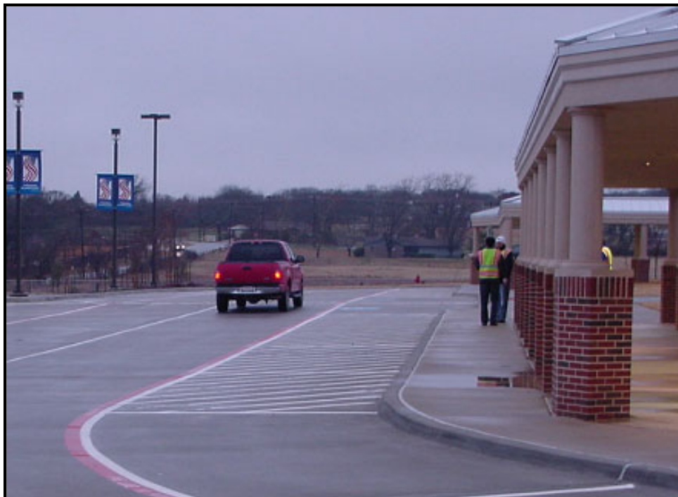
Figure 18. Covered Walkway Adjacent to the Parent Loading Zone.
