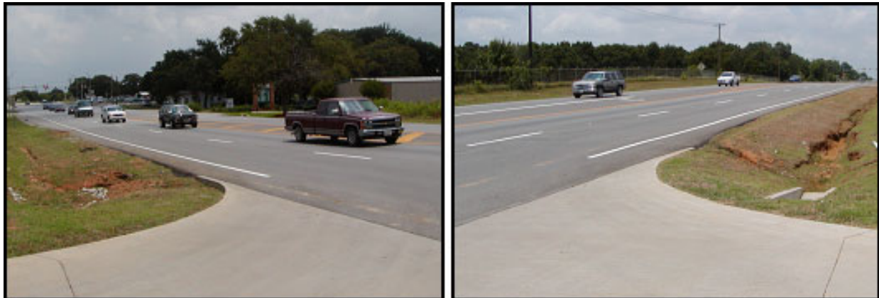
Figure 13. Good Example of School Driveway with Good Sight Distance in Both Directions.
