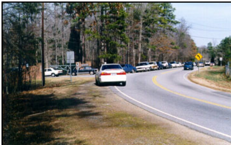
Figure 51. Traffic Queue on Unpaved Shoulder – Right-Turn Lane Might Be Warranted.
