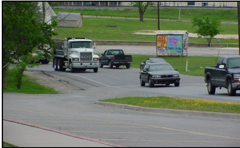
Figure 14. Site with Driveway Located near Horizontal Curve – Inadequate Sight Distance.
