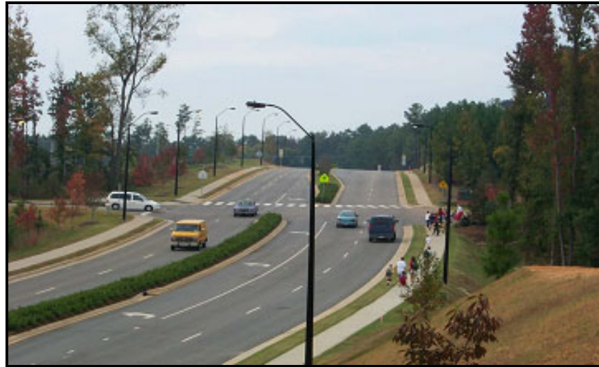
Figure 39. Roadway near School with Well-Maintained Sidewalks on Both Sides of Street.
