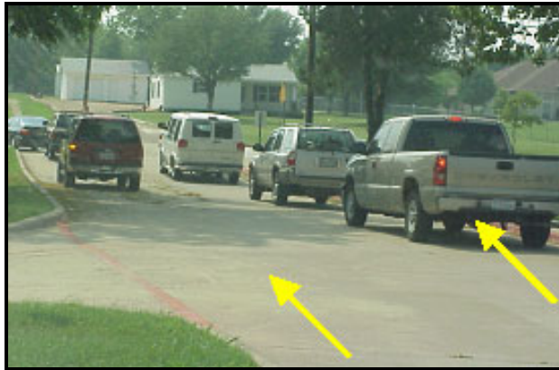
Figure 50. School Exit Driveway with Two Lanes for Left and Right Turn Movements.
