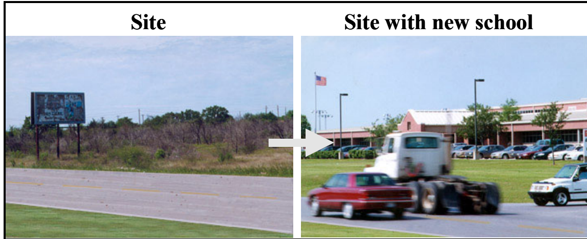
Figure 10. School Site Located on High-Speed Roadway without Turn Lanes.
