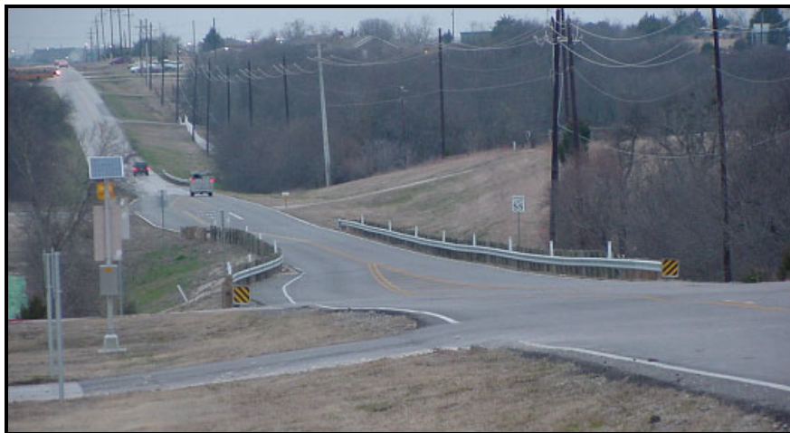
Figure 40. School Site Located on Two-Lane High-Speed Roadway – No Sidewalks.
