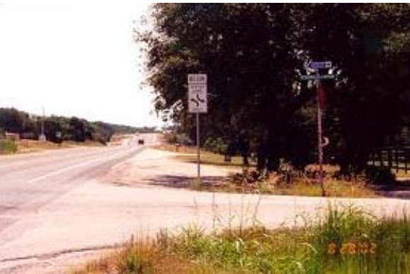
Figure 4-13. At PCT Intersection Facing EB.
