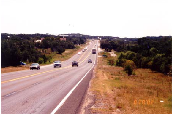
Figure 4-11. Eastbound with PCT on the Right (second drive).
