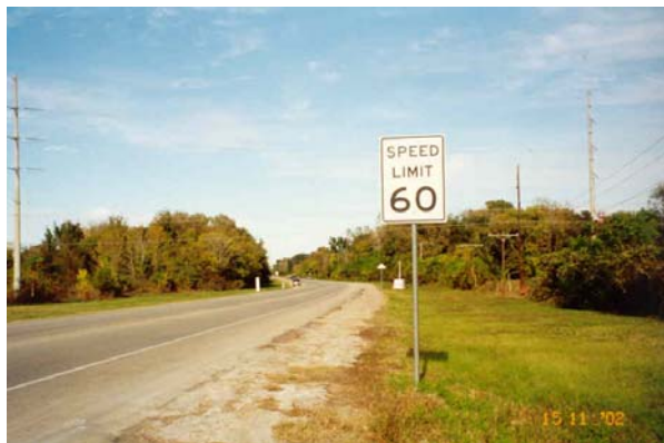
(a) Just Downstream of Intersection
