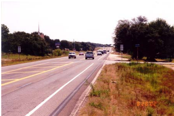
Figure 4-12. Looking EB as Vehicle Turns Left onto PCT Using TWLTL.
