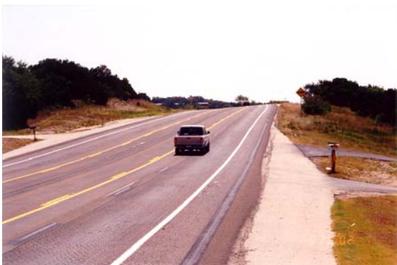
Figure 4-15. EB toward Austin Showing Grade.
