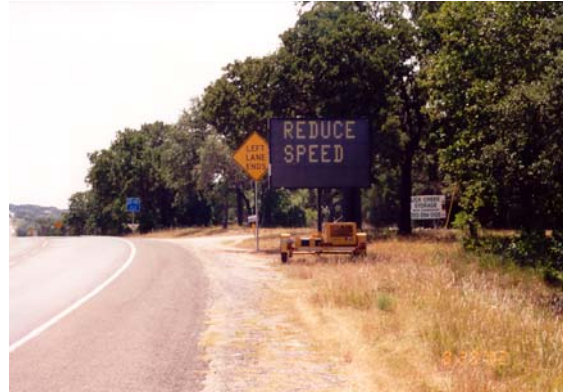
Figure 4-9. Changeable Message Sign and Sign Showing Changes to Roadway.
