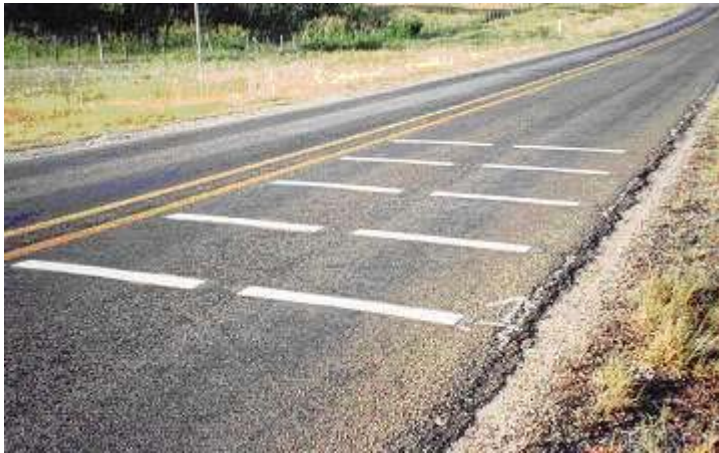
(a) Set of In-Lane Rumble Strips.
