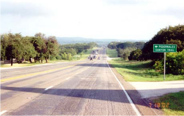
Figure 4-4. Looking West toward PCT Intersection (about halfway into picture on left side).
