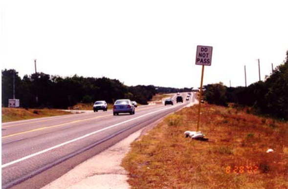
Figure 4-14. Do Not Pass Sign, Looking East, Video Trailer on Left.
