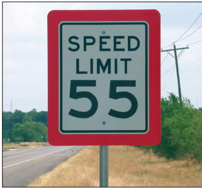
Figure 4. 3-Inch Red Microprismatic Border on Speed Limit Sign.
