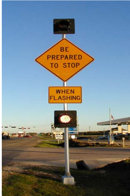
a. Pole-mounted AWECS Advance Traffic Control Sign (W3-4) near Waco.
