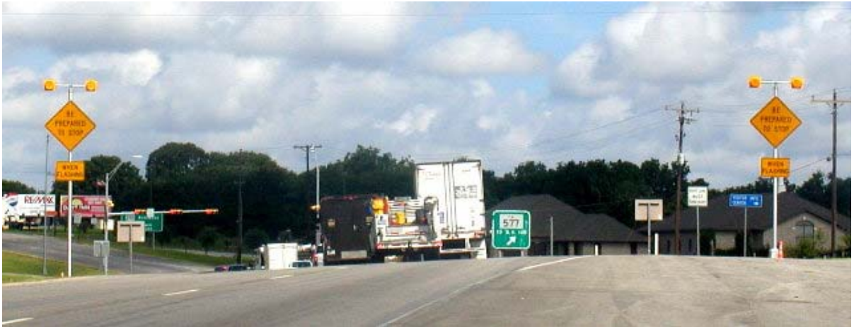
b. Two Pole-mounted AWECS Advance Traffic Control Signs (W3-4) in Brenham.
