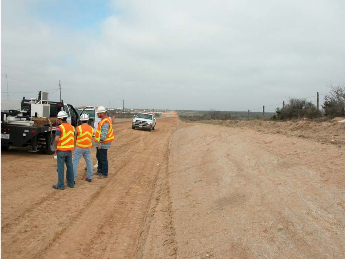
Figure 22. FM 3338 is an 8-Mile Long Widening Project in the Laredo District.
