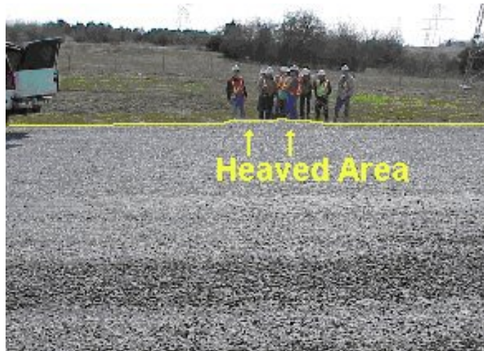
Figure 4. Heaved Area on the Eastbound Side of US 82 Near Sherman, Texas.
