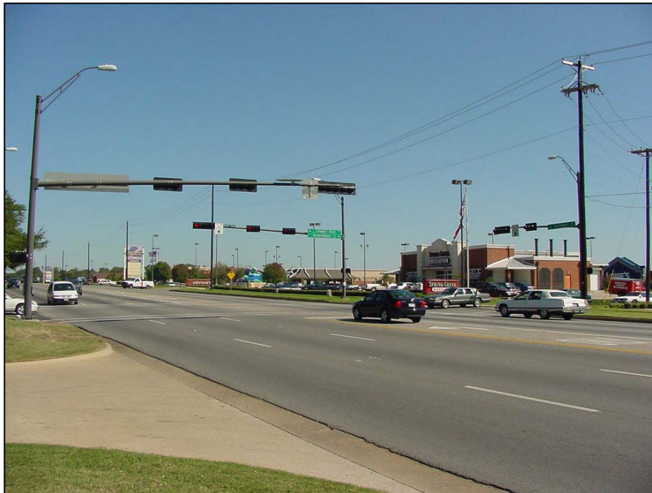
Figure 2-10. Broadway Avenue Facing North to Chimney Rock Signalized Intersection.
