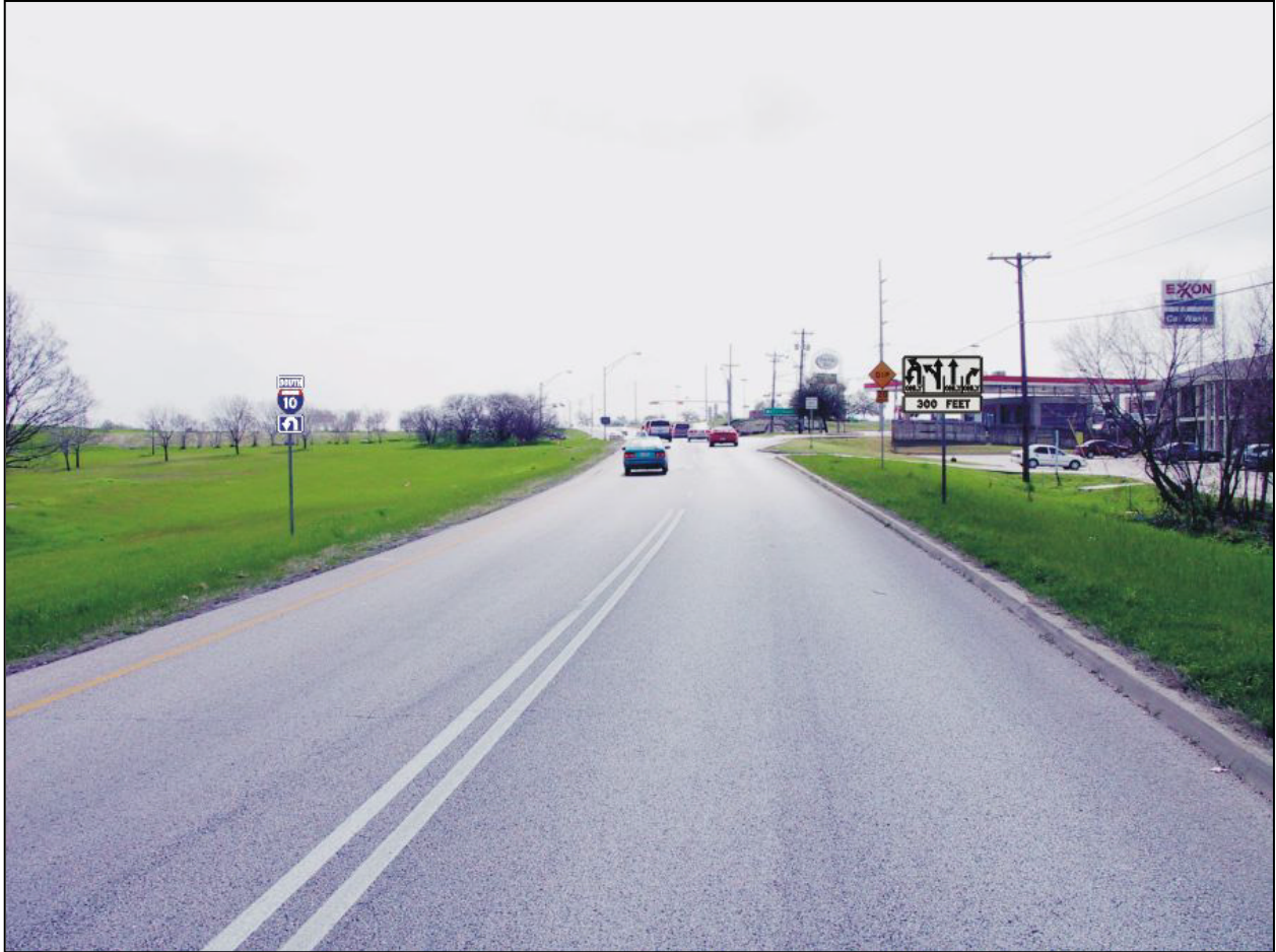
Figure 14. Frontage Road with Complex Lane Assignment Sign.
