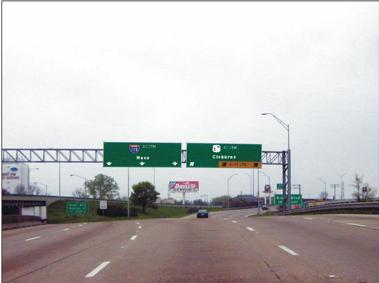
Figure 11. Freeway Split with Downward Pull-Through Arrows for the Through Lanes and Diagonal Up Arrows for Exiting Lanes.
