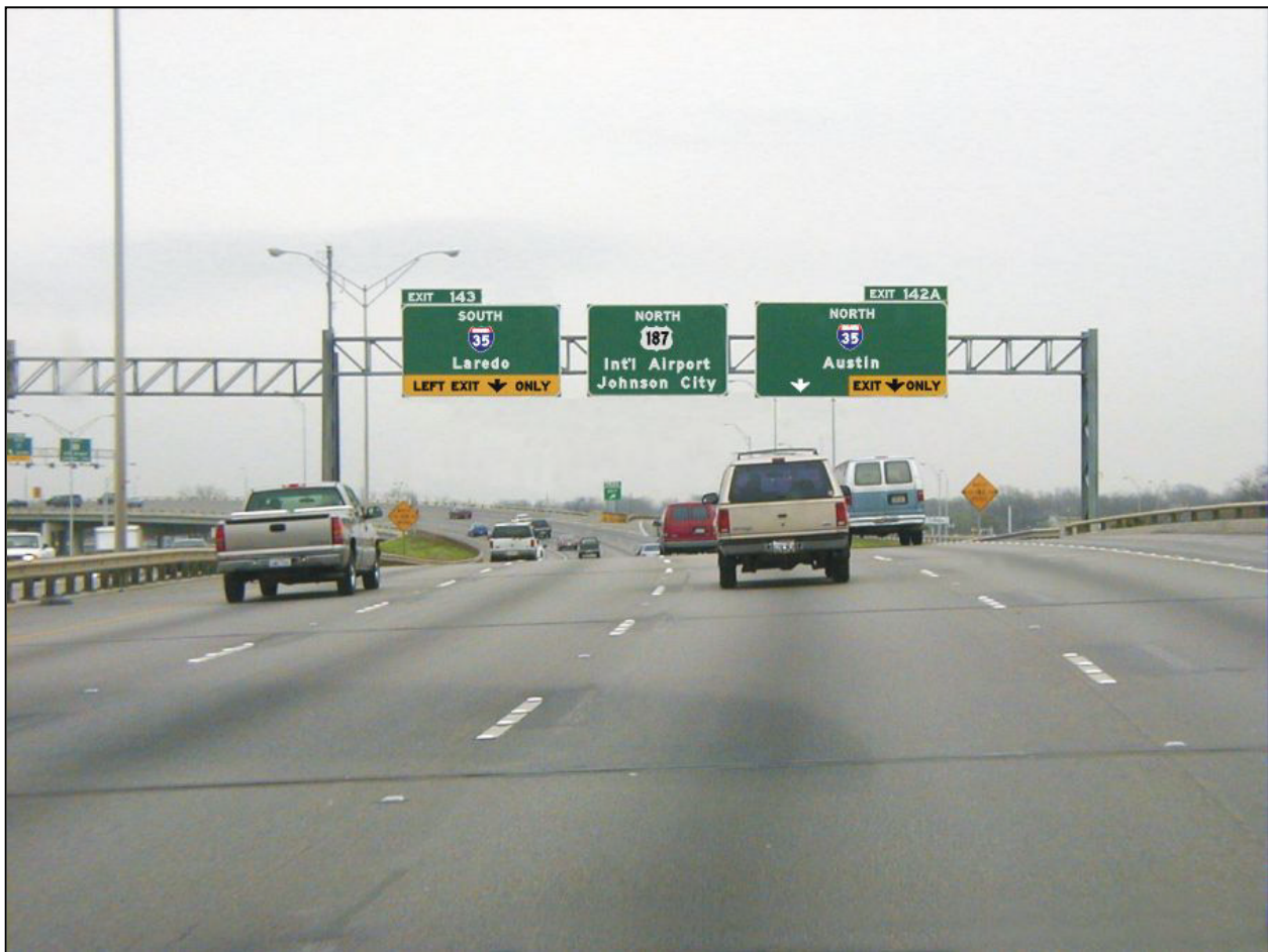
Figure 7. Addition of the Word “LEFT” to the EXIT ONLY Panel.
