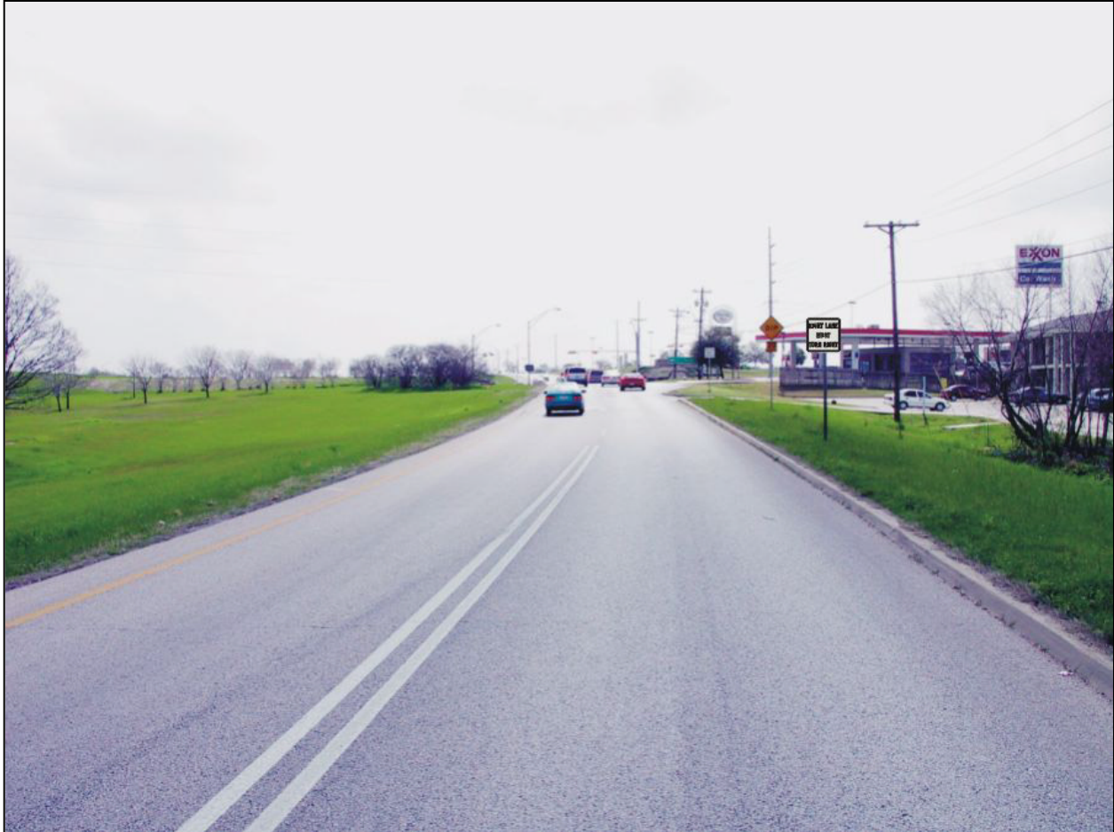
Figure 12. Frontage Road Sign with RIGHT LANE MUST TURN RIGHT Sign.
