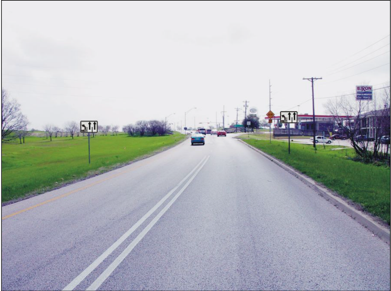
Figure 13. Frontage Road with Symbol Lane Assignment Sign.
