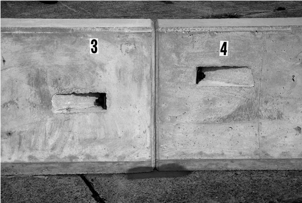
Figure 11. Cross-Bolt, F-Shape Precast Concrete Traffic Barrier before Test 441623-1.
