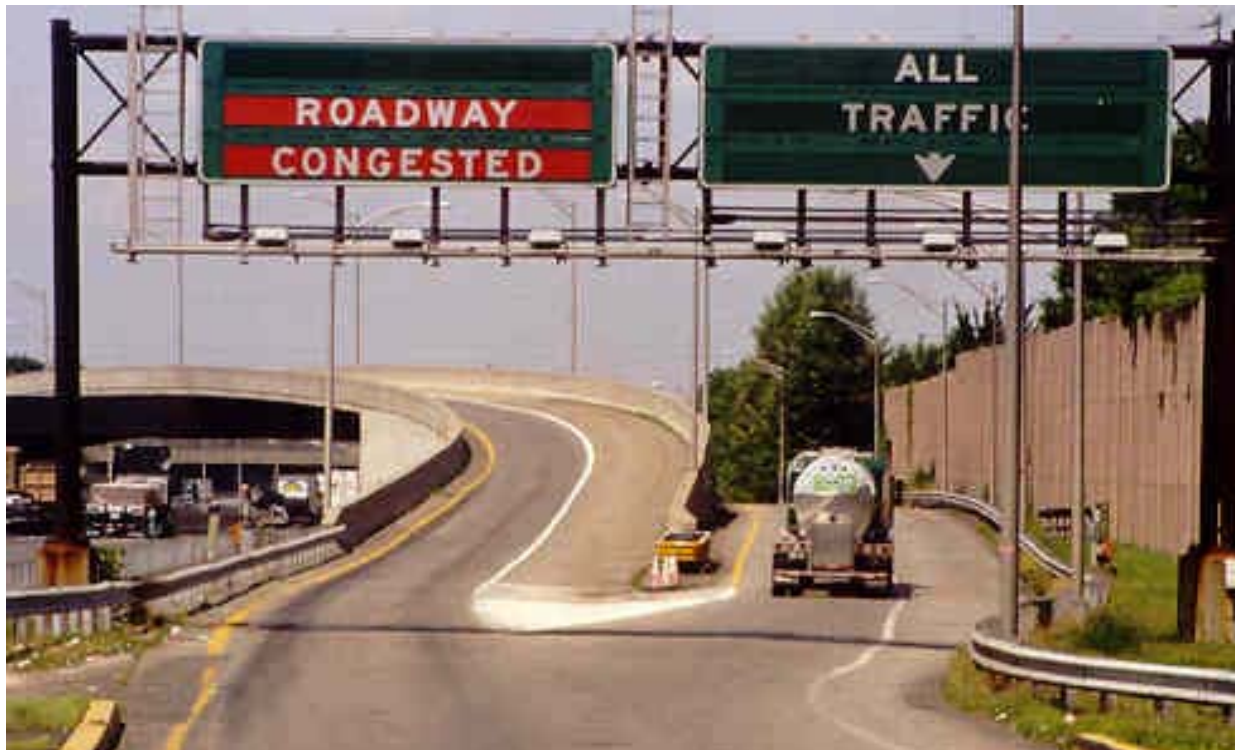
Figure 3-4. Entrance Ramp to the Dual-Dual Roadway of the New Jersey Turnpike.
