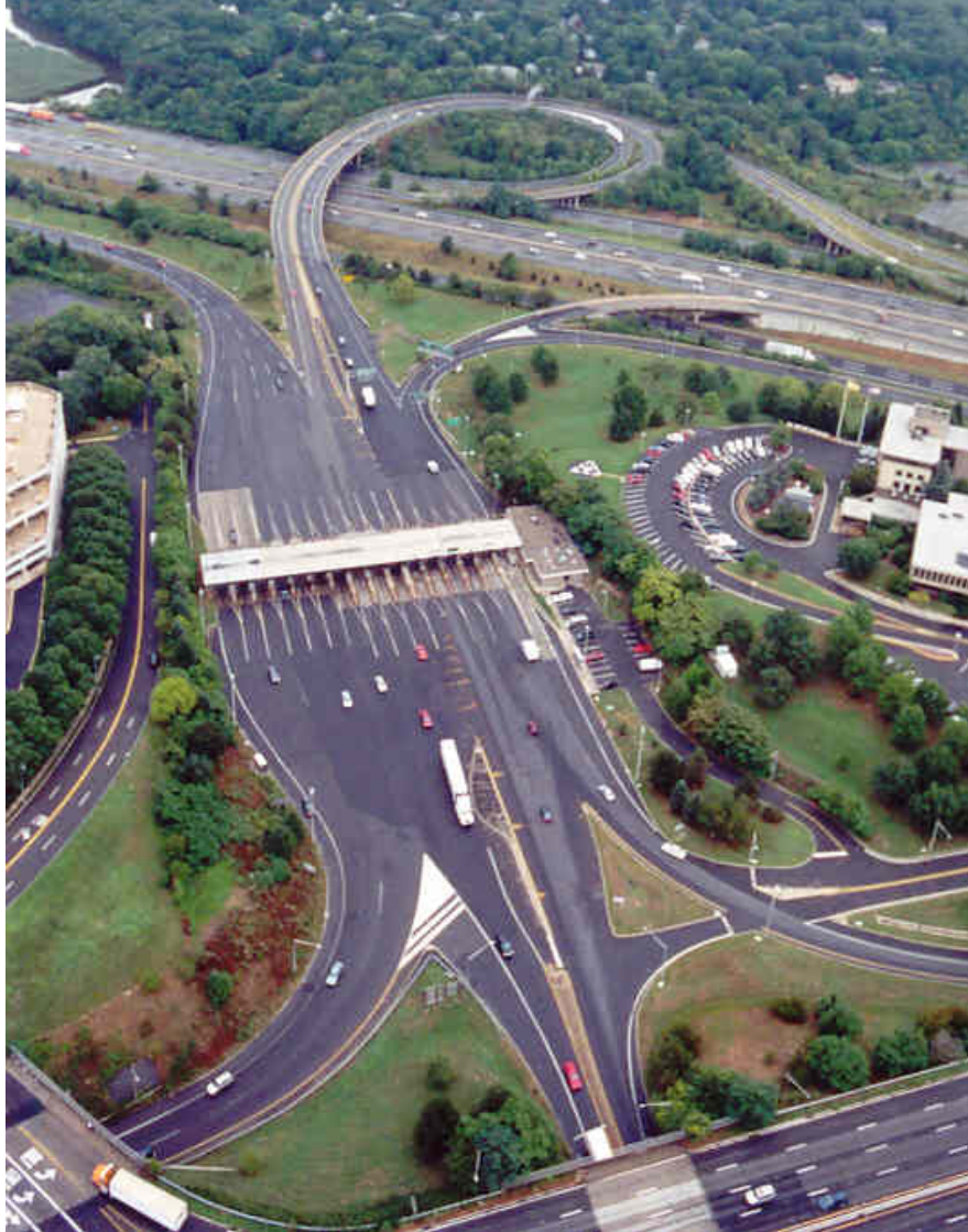
Figure 3-6. New Jersey Turnpike Toll Plaza.
