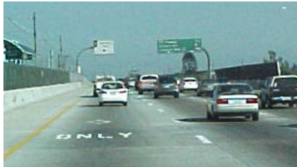
Figure 21. Example of Cantilevered Signs in California.
