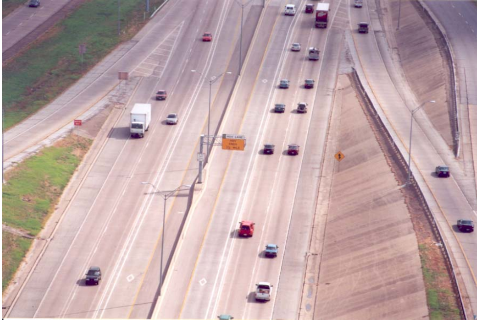
Figure 25. HOV Lane Pavement Marking Symbols in Houston.
