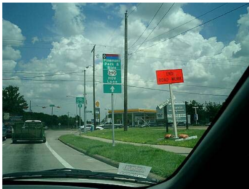
Figure 20. Trailblazer Sign on Suburban Arterial in Houston.
