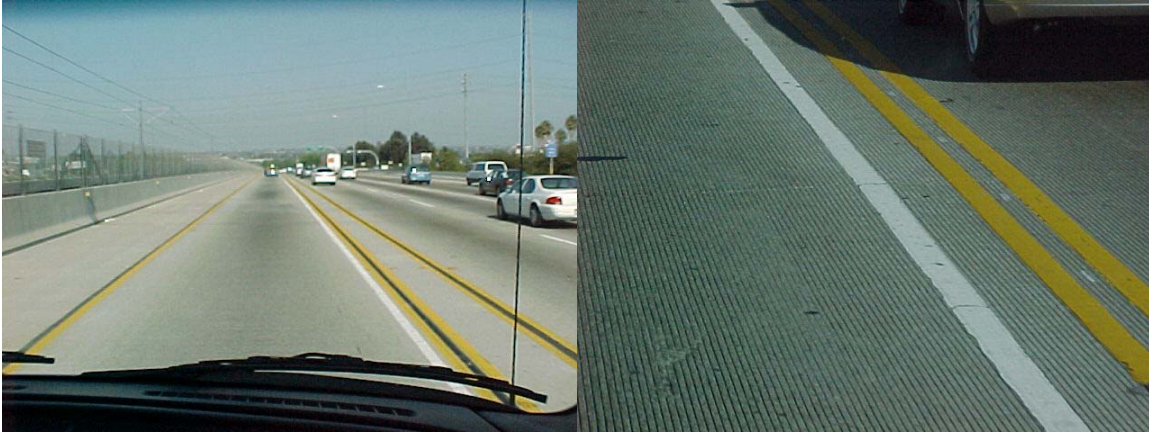
Figure 24. Yellow Lane Lines Used in California.
