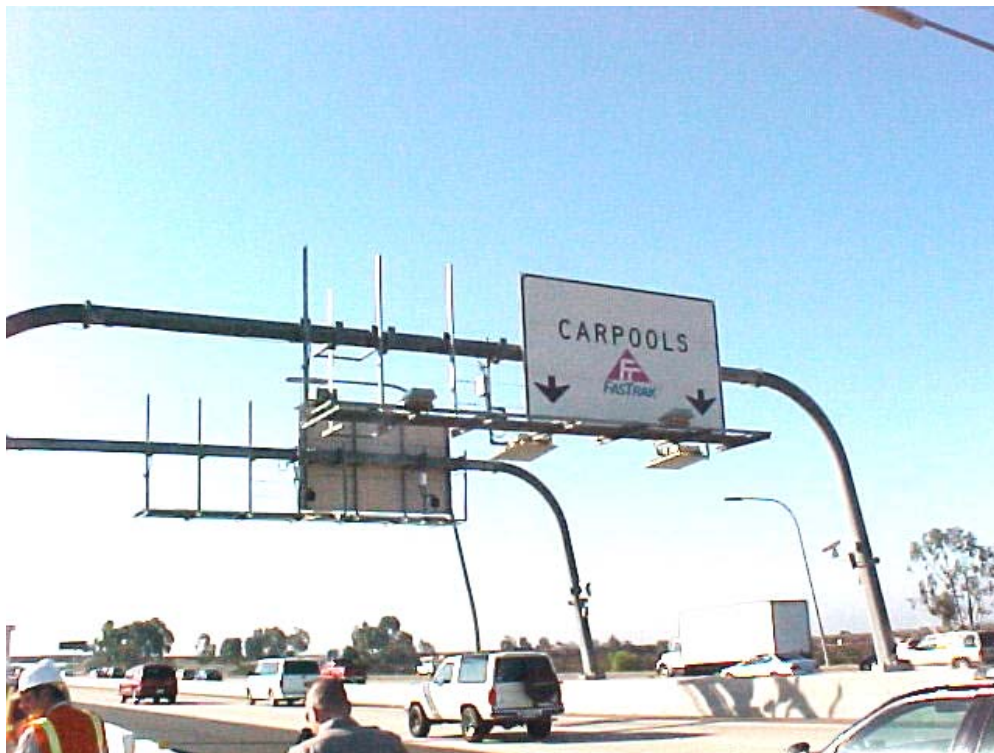
Figure 8. HOT Lane on I-15 in San Diego.
