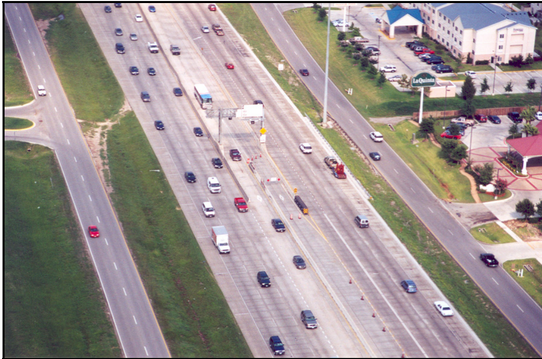
Figure 6. Example of a Reverse Flow Barrier-Separated Facility (photo taken in Houston).
