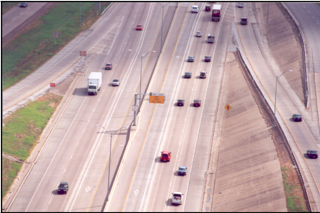
Figure 5. Example of a Concurrent Flow Buffer-Separated Facility (photo taken in Dallas).
