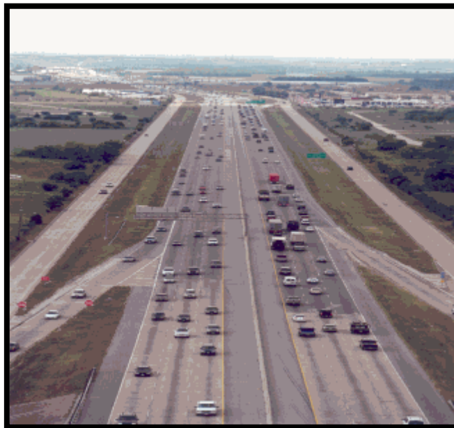
Figure 3-1. Freeway with Frontage Roads.
