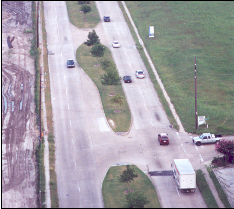
Figure 2-16. Full Median Opening (undeveloped area) in Houston, Texas.
