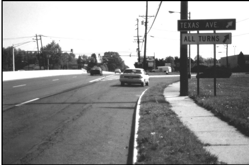
Figure 2-23. Upstream (Near Side) Jughandle Configuration.
