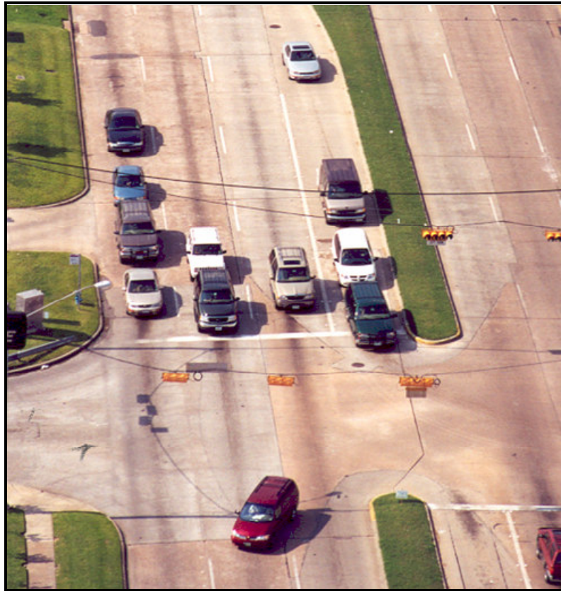
Figure 2-12. Insufficient Corner Clearance.
