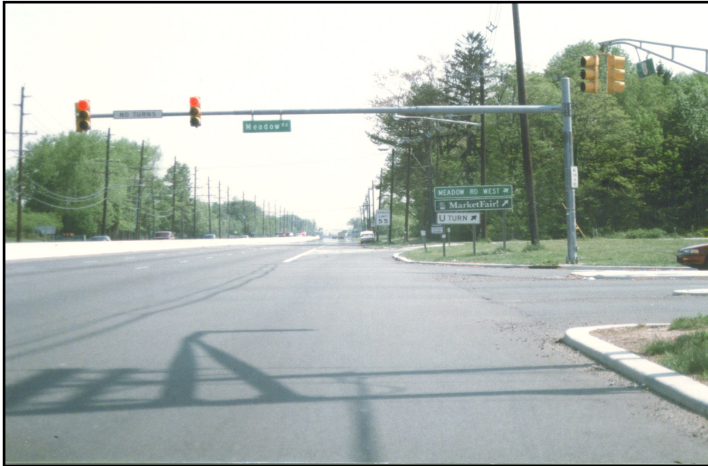
Figure 2-24. Downstream (Far Side) Jughandle Configuration.
