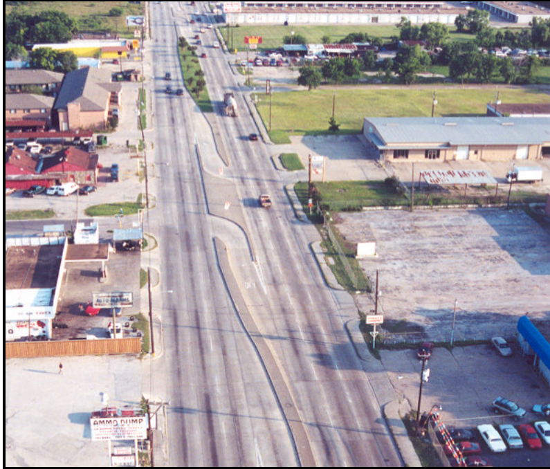
Figure 2-14. Directional Median Opening in Houston, Texas.
