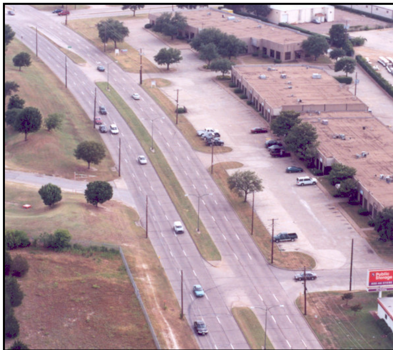
Figure 2-9. Unsignalized Access in Dallas, Texas.
