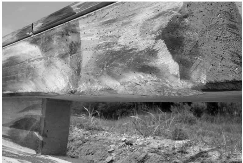
Figure B-9. Installation after Test 441382-2.
