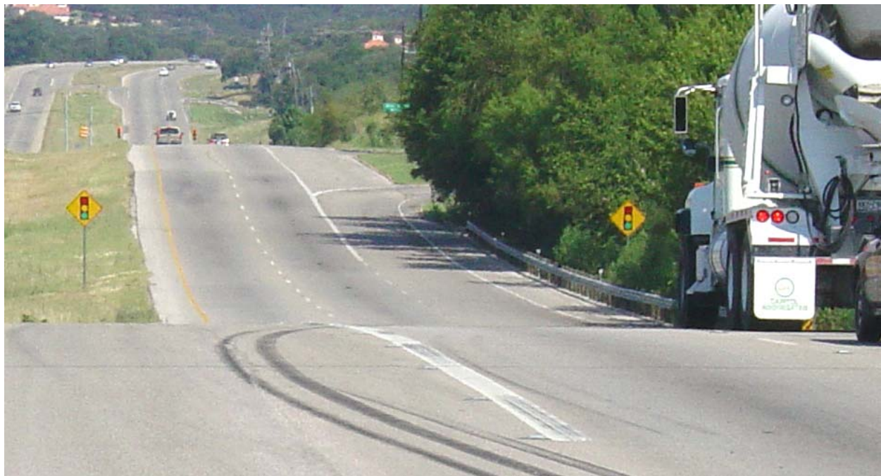
Figure 27. Study Signing (Dual Symbolic SIGNAL AHEAD Signs) Installed at Site 1.
