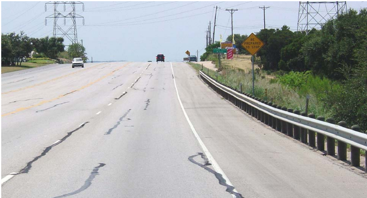
Figure 29. Study Signing (BE PREPARED TO STOP) Installed at Site 2.
