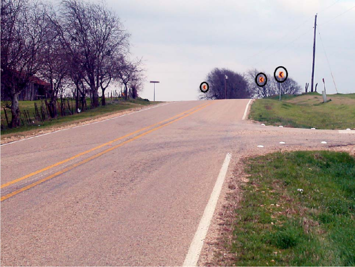
Figure 5. Another Example of Chevrons along a Curve.
