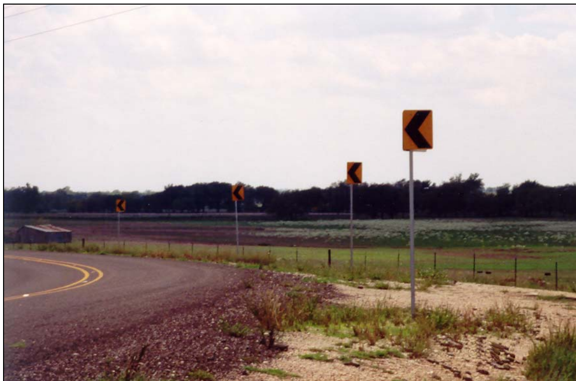
Figure 5-10. Chevrons on Horizontal Curve.
