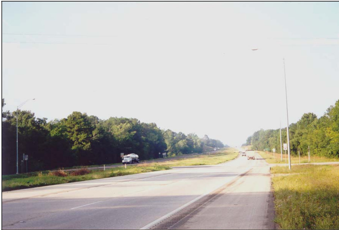
Figure 4-4. Safety Lighting at Site 99-06.
