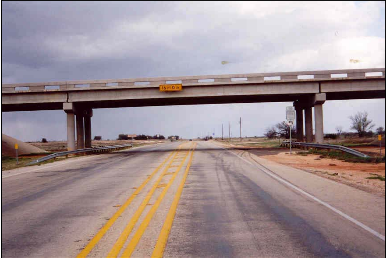
Figure 3-16. View of Grade Separation Structure at Site 98-05.
