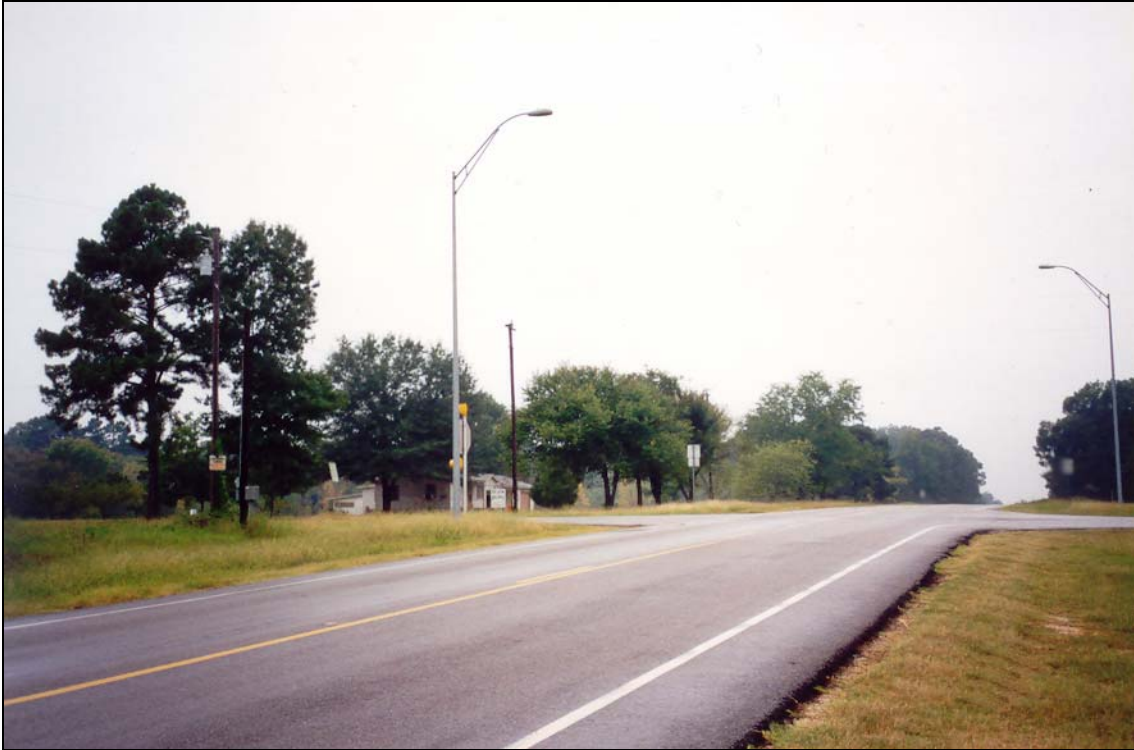
Figure 5-8. Luminaires on Opposite Corners of Four-Leg Intersection.
