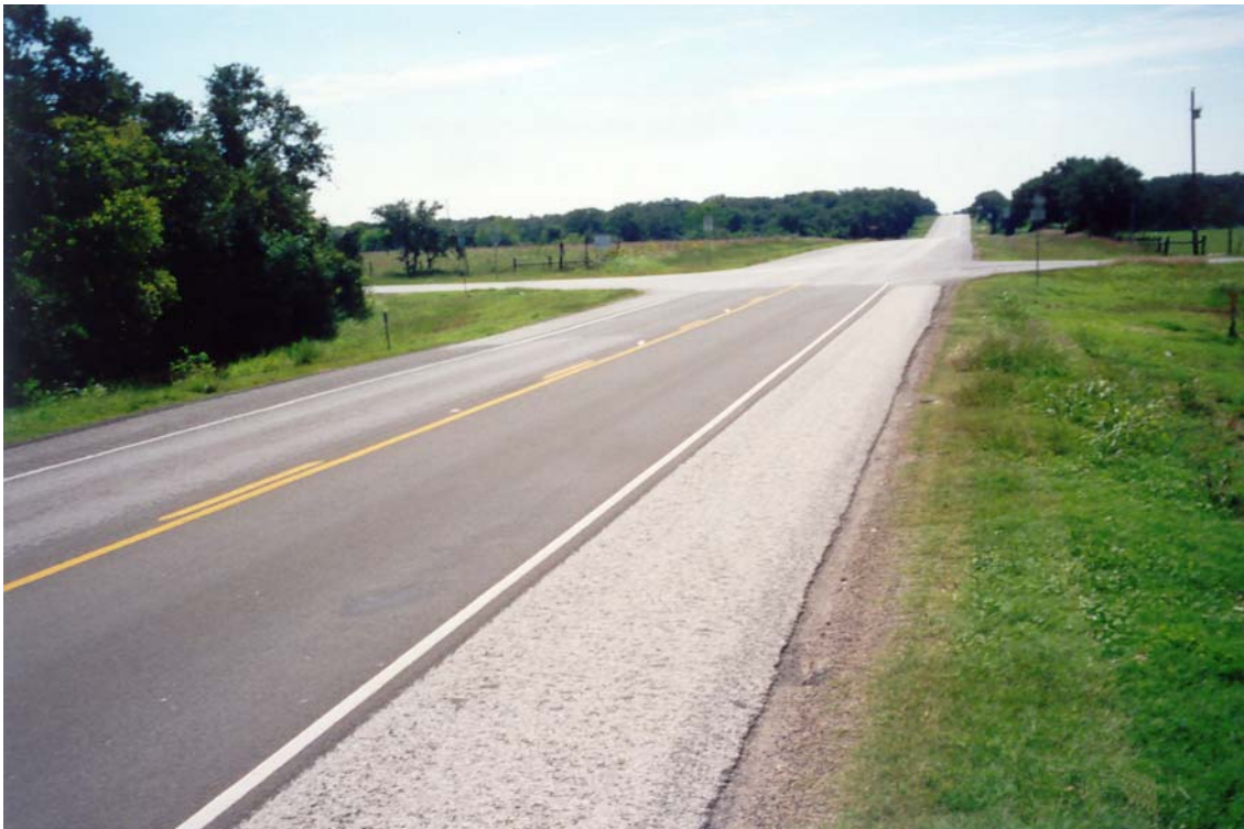
Figure 5-5. View of Resurfaced Roadway and Added Shoulders at Site 100-06.
