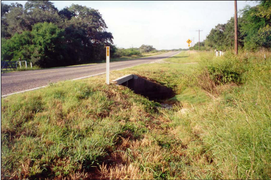
Figure 4-6. Improvements at Site 99-08.
