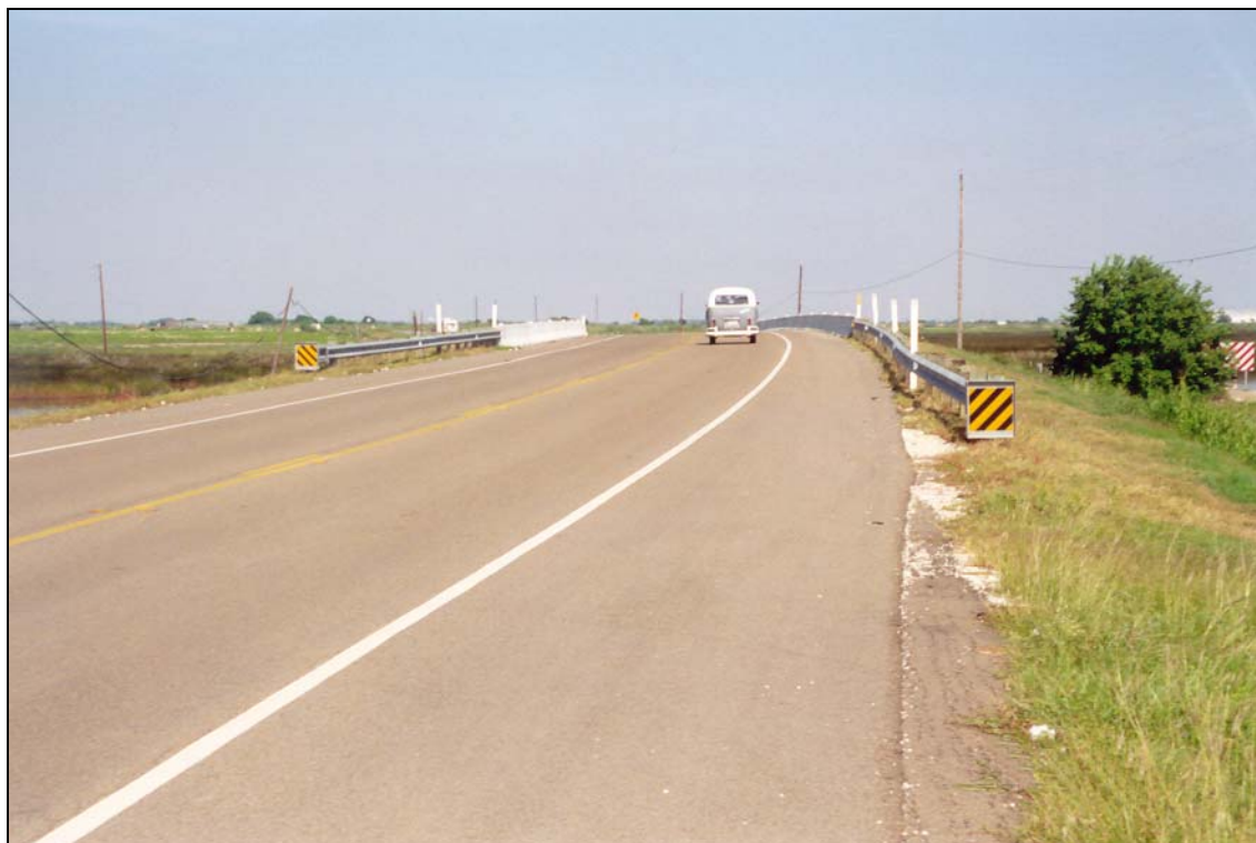
Figure 4-3. Added Shoulders, Resurfacing, and Safety Treatments.
