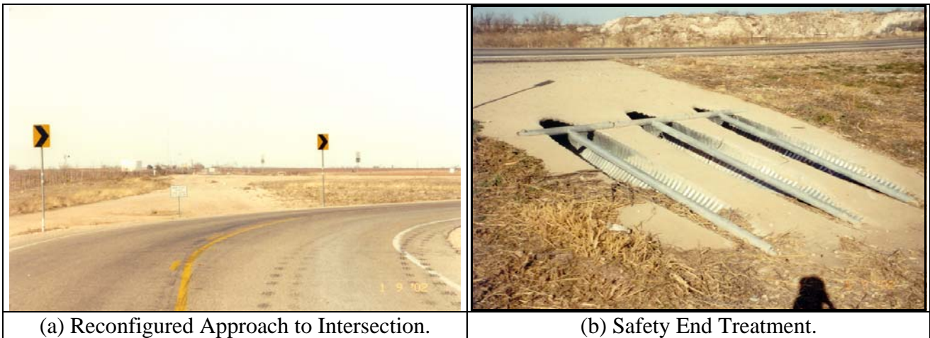
Figure 4-2. Improvements at Site 99-04.
