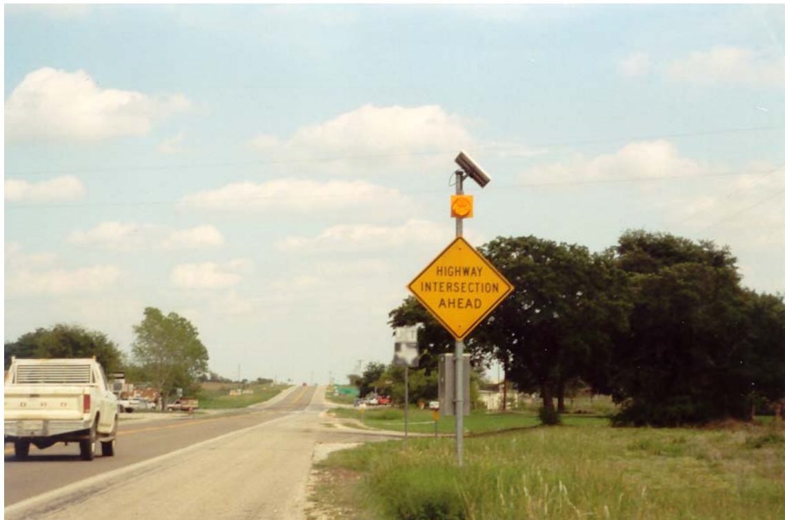
Figure 4-7. Advance Warning Sign with Flashing Beacons on Obscured Approach.
