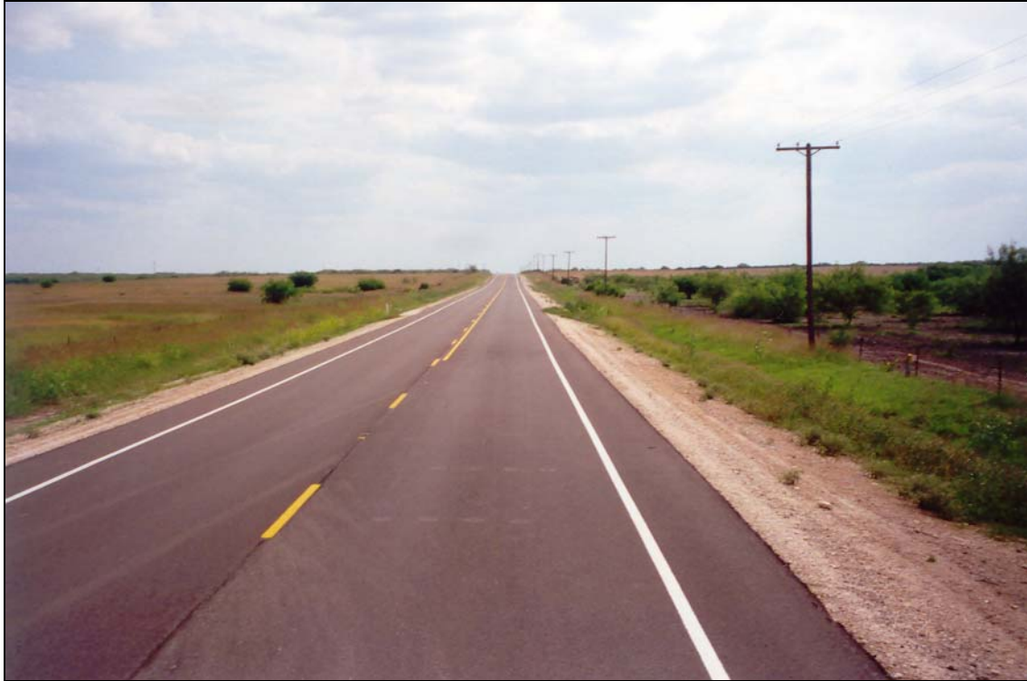
Figure 5-4. Widened Roadway at Site 100-05.
