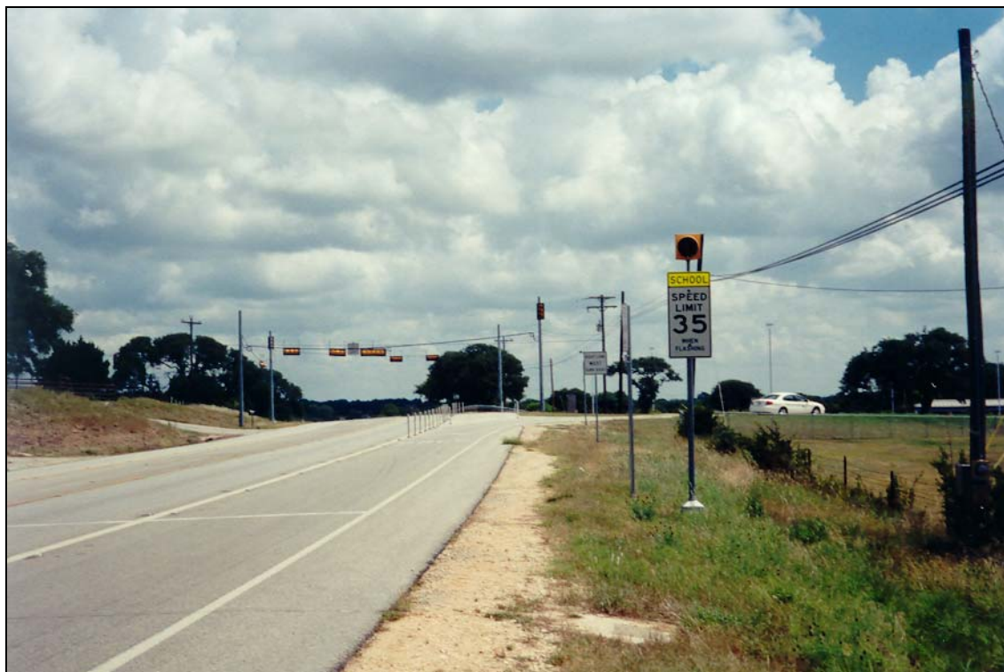
Figure 5-16. Right-Turn Lane Adjacent to School.
