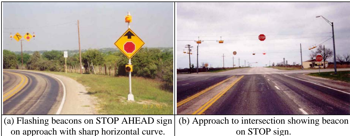
Figure 3-12. Improvements at Site 98-01.
