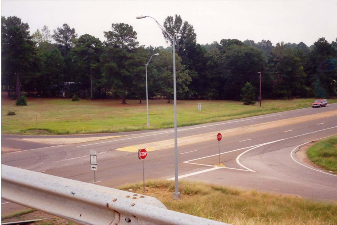
Figure 5-6. Safety Lighting at Site 100-07.
