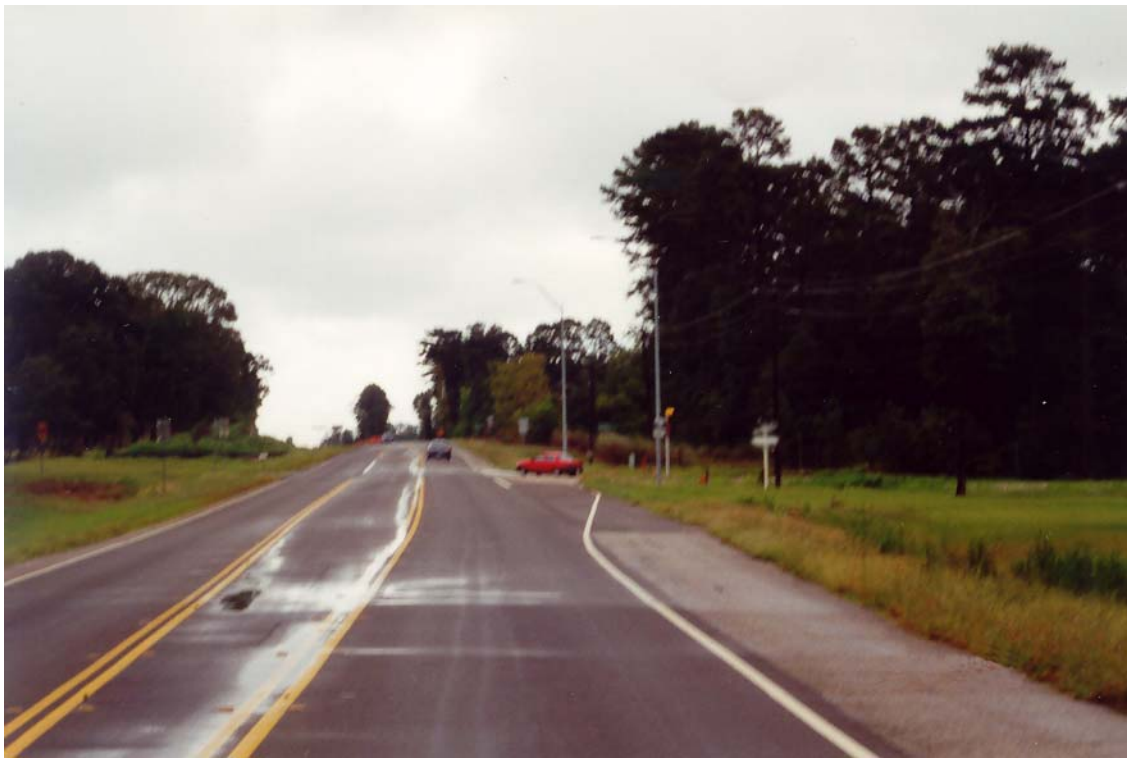
Figure 5-7. Luminaires at T-Intersection.
