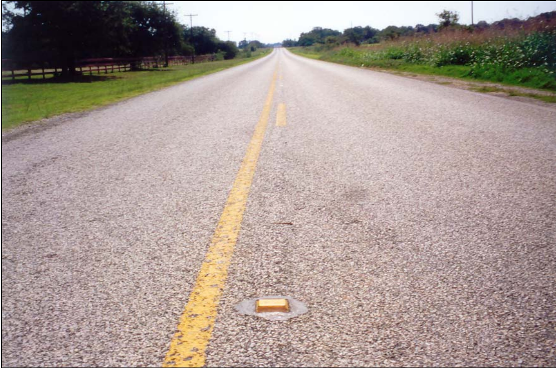
Figure 5-13. Centerline Raised Pavement Marker.
