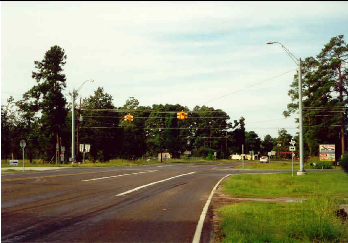
Figure 3-21. View of Safety Lighting at Site 98-10.
