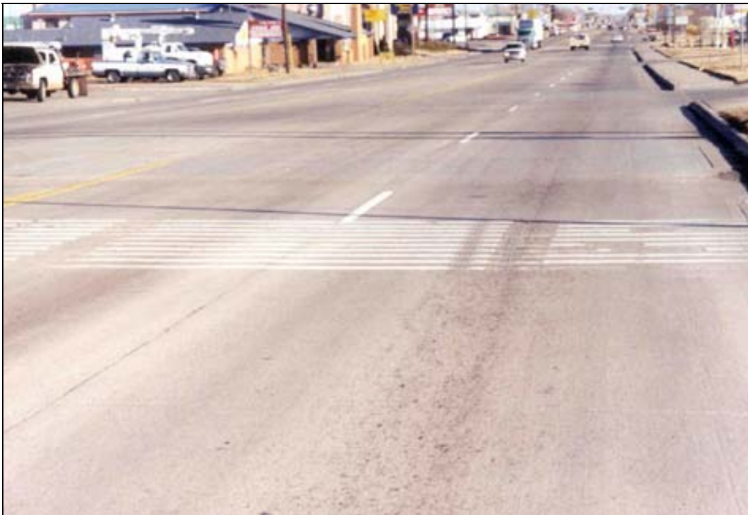
Figure 3-7. View of Approach Rumble Strips.
