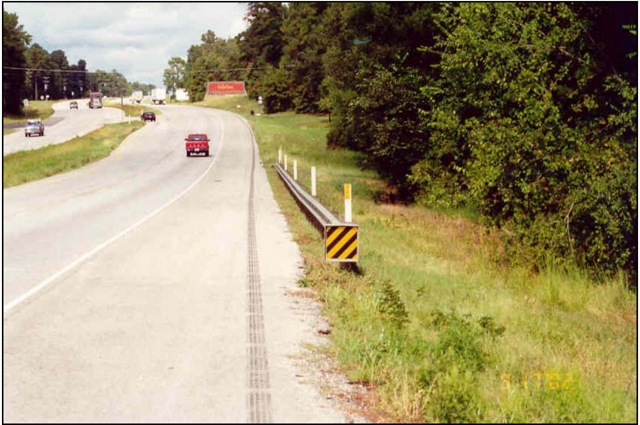
Figure 3-11. Safety Treated Guardrail.
