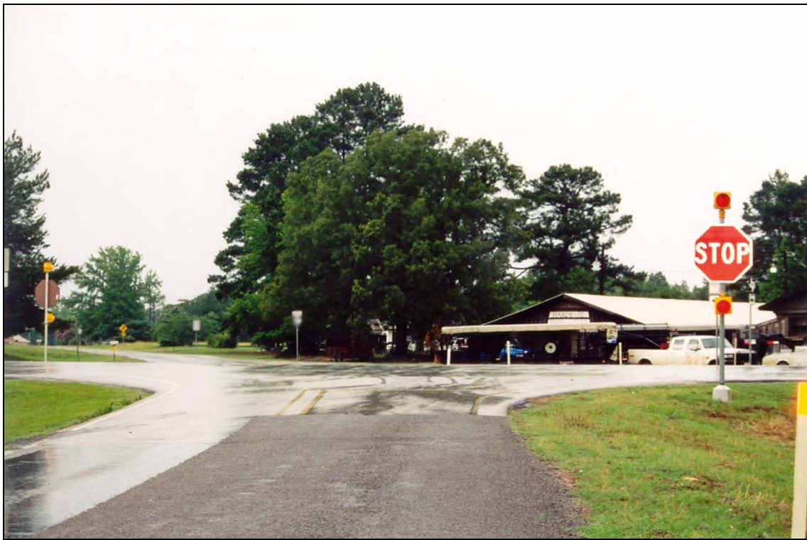
Figure 4-8. Beacons Mounted on STOP Sign.
