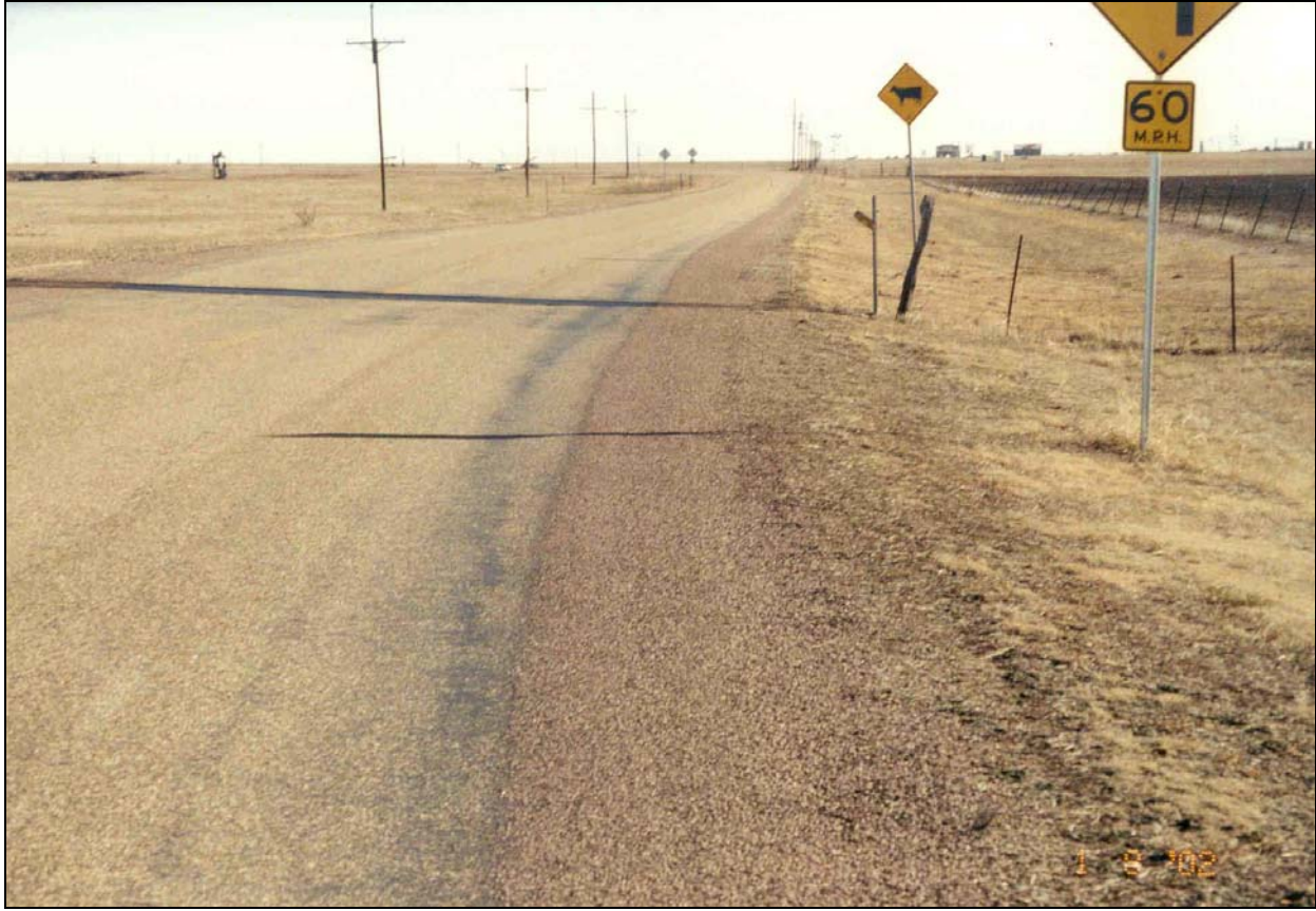
Figure 3-10. View of Roadway Widening.
