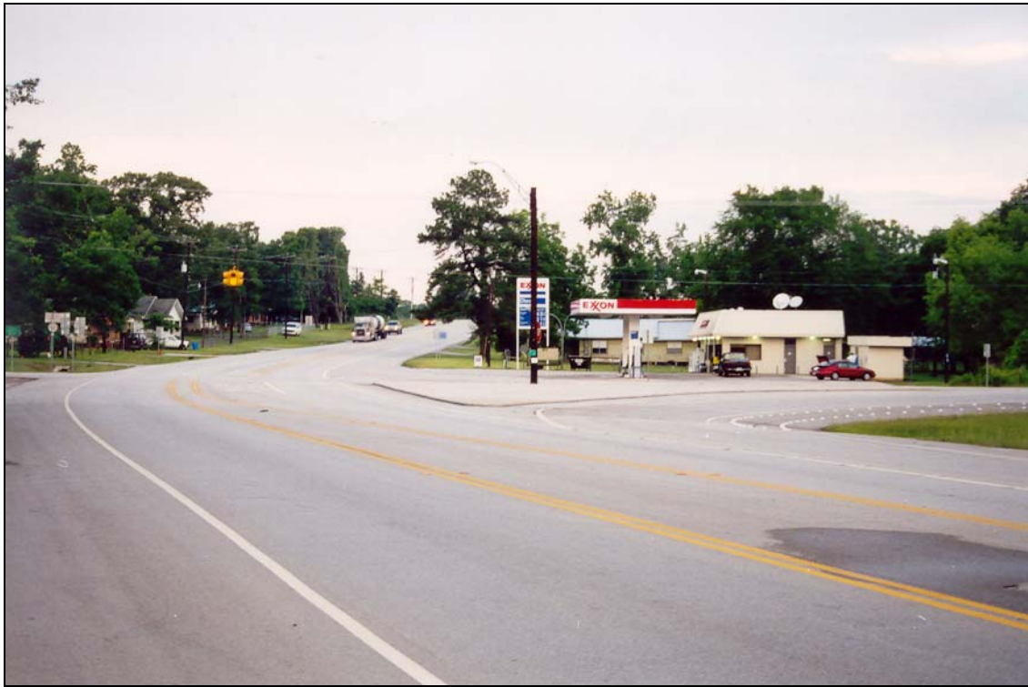
Figure 5-18. Right-Turn Lane with Channelizing Island.
