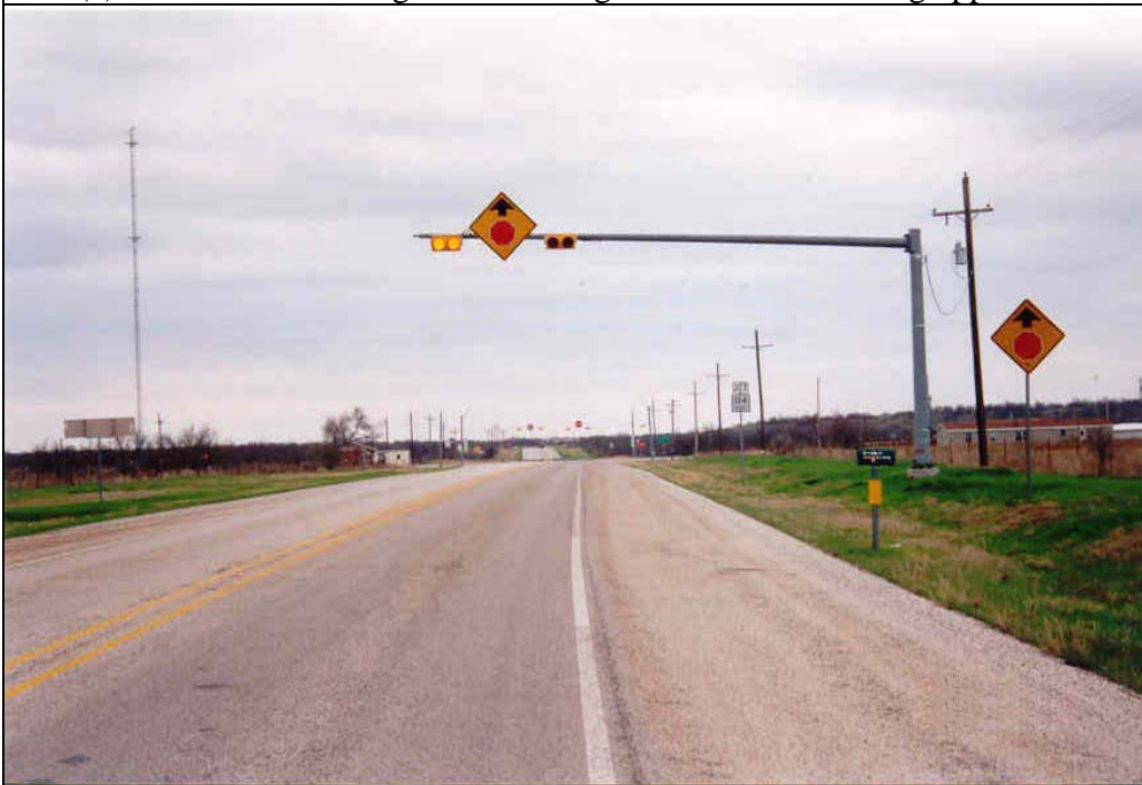
(b) Overhead advance warning flashers and additional STOP AHEAD sign on minor approach.
