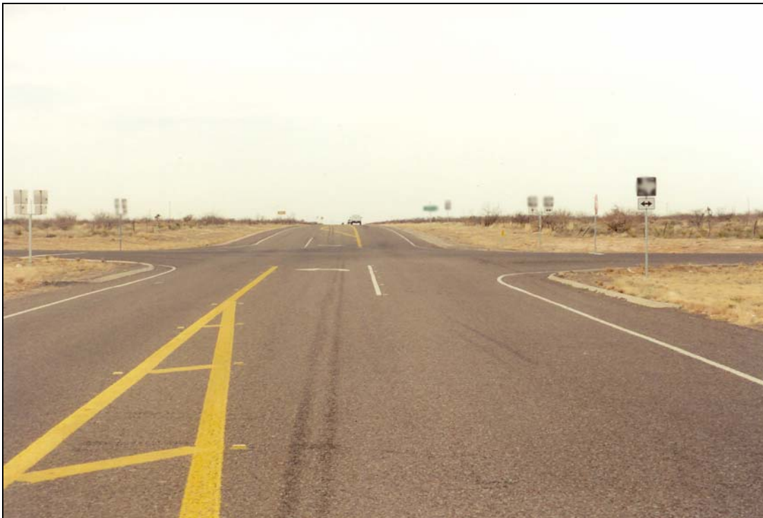
Figure 5-12. New Left-Turn Lanes at Intersection.
