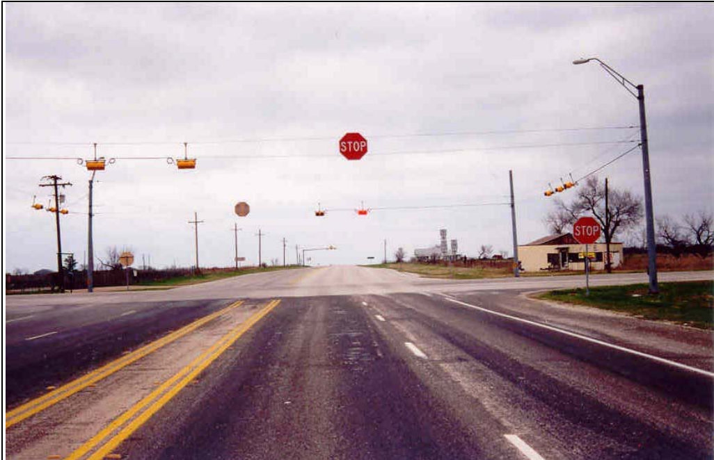
(a) Overhead STOP sign and flashing beacons on minor leg approach.
