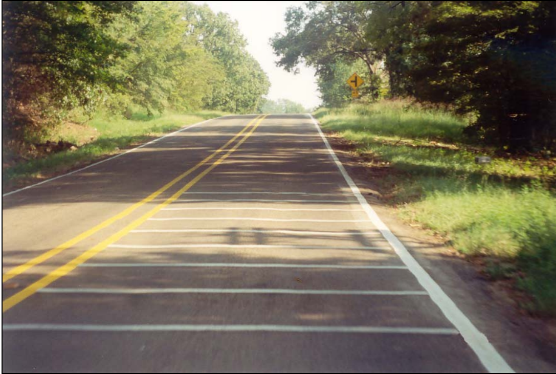
Figure 5-14. Approach Rumble Strips and Intersection Advance Warning Sign.
