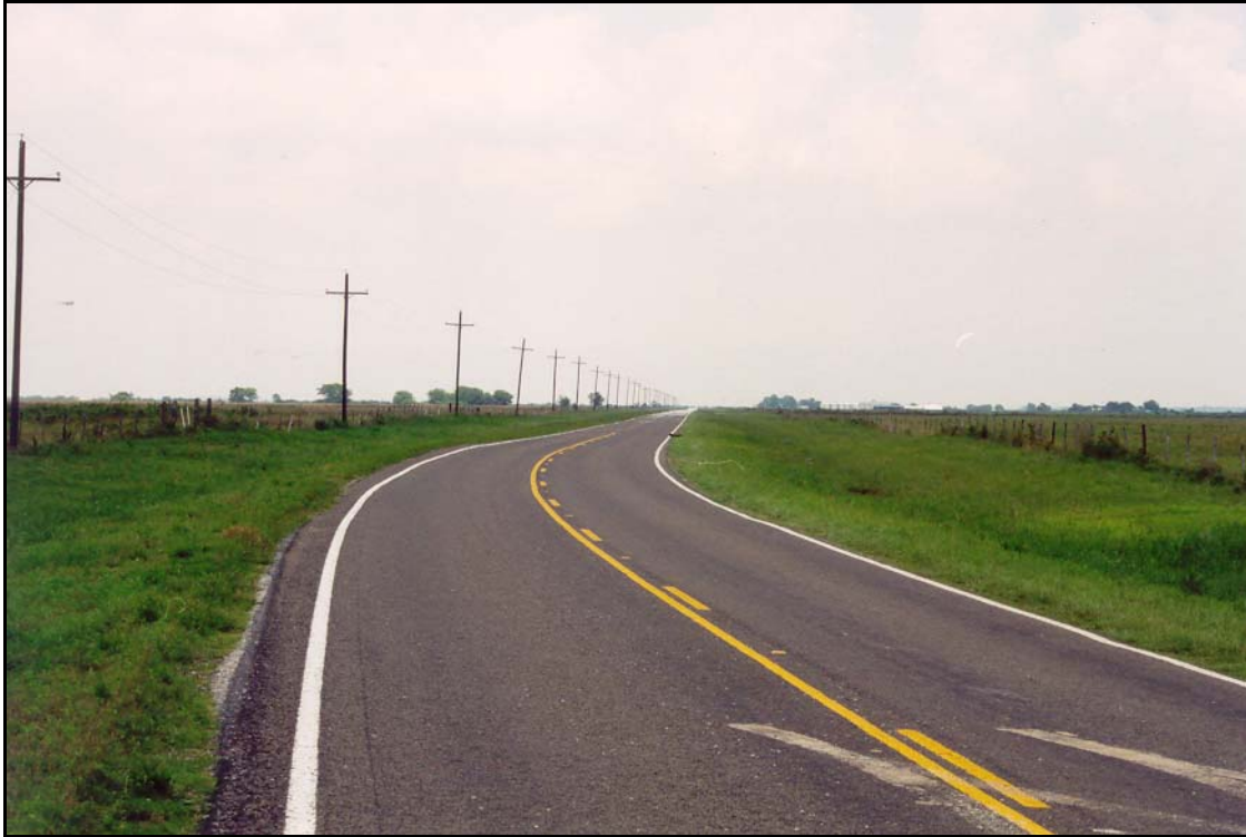
Figure 5-20. Widened Lanes at Site 100-24.
