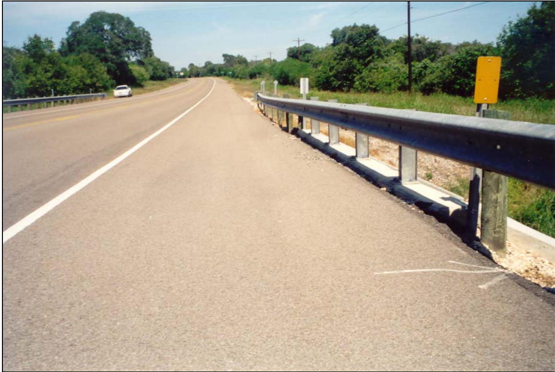
Figure 5-1. New Shoulders and Resurfacing at Site 100-02.
