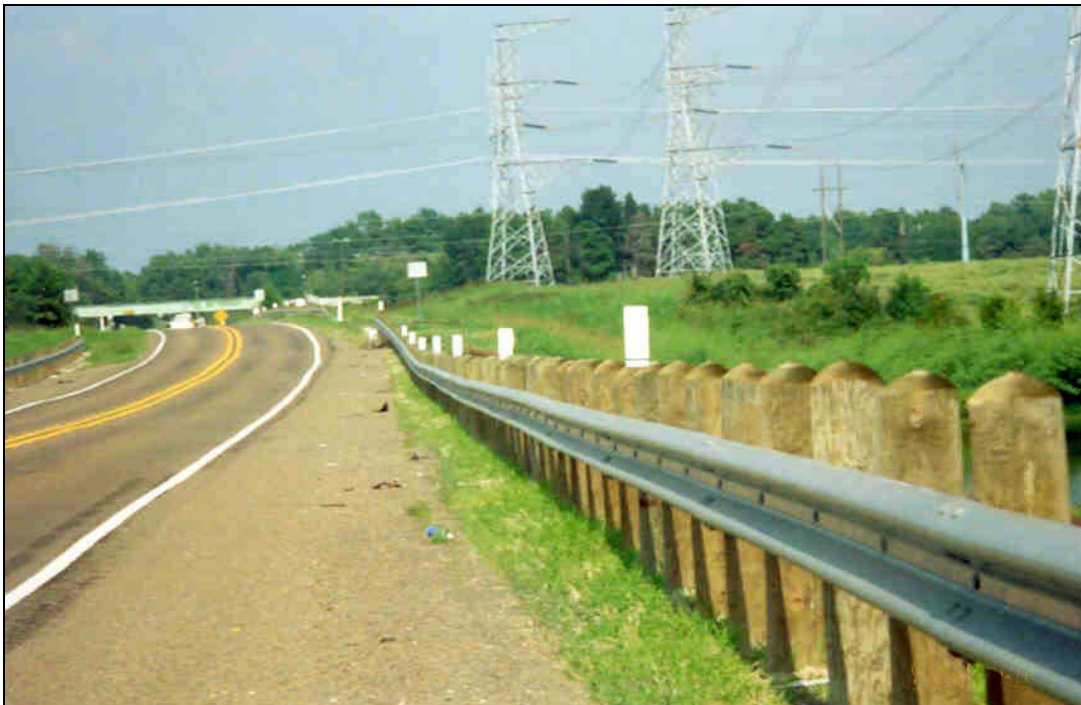
Figure 3-4. View of Added Raised Pavement Markers and Delineation.
