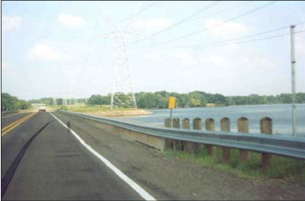
Figure 3-3. View of Bridge on Lake.
