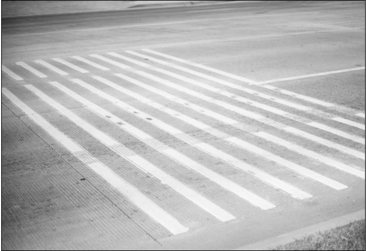
Figure 3-9. Close-Up View of Approach Rumble Strips.
