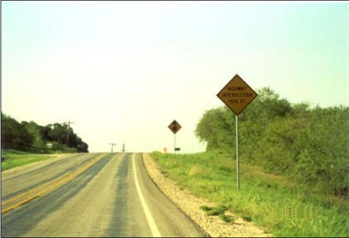
Figure 3-6. Advance Warning Signs for Approach to Intersection.
