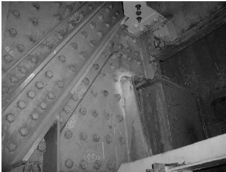
Figure 108. Diagonal Rib Installed to Improve Load Path.
