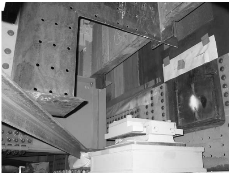
Figure 111. Dap End Removed; New Support in Place for Straight Beam.
