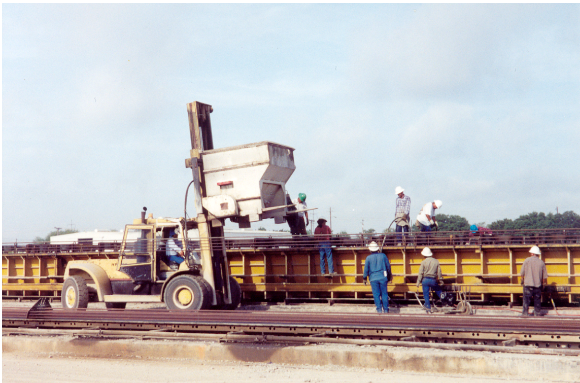
Figure 2.2. Transportation and Placement of Concrete for Girders.
