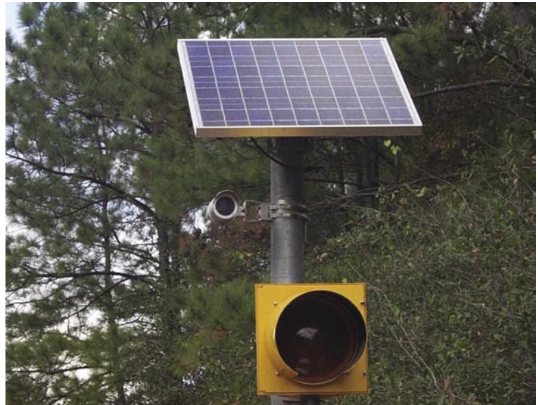
Figure 1. Flashing beacon assembly
