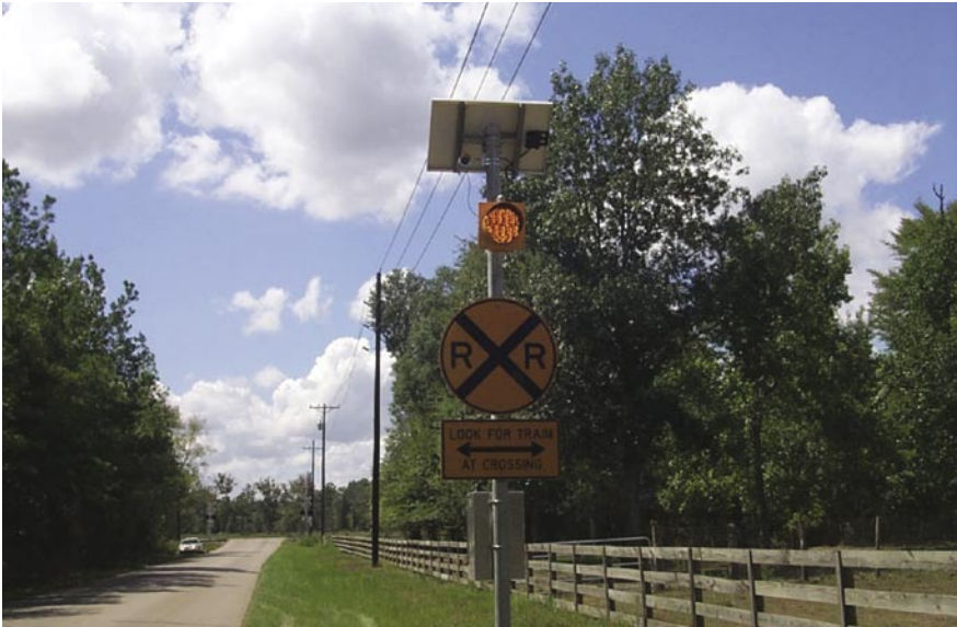
Figure 3. Site conditions determined sign location
