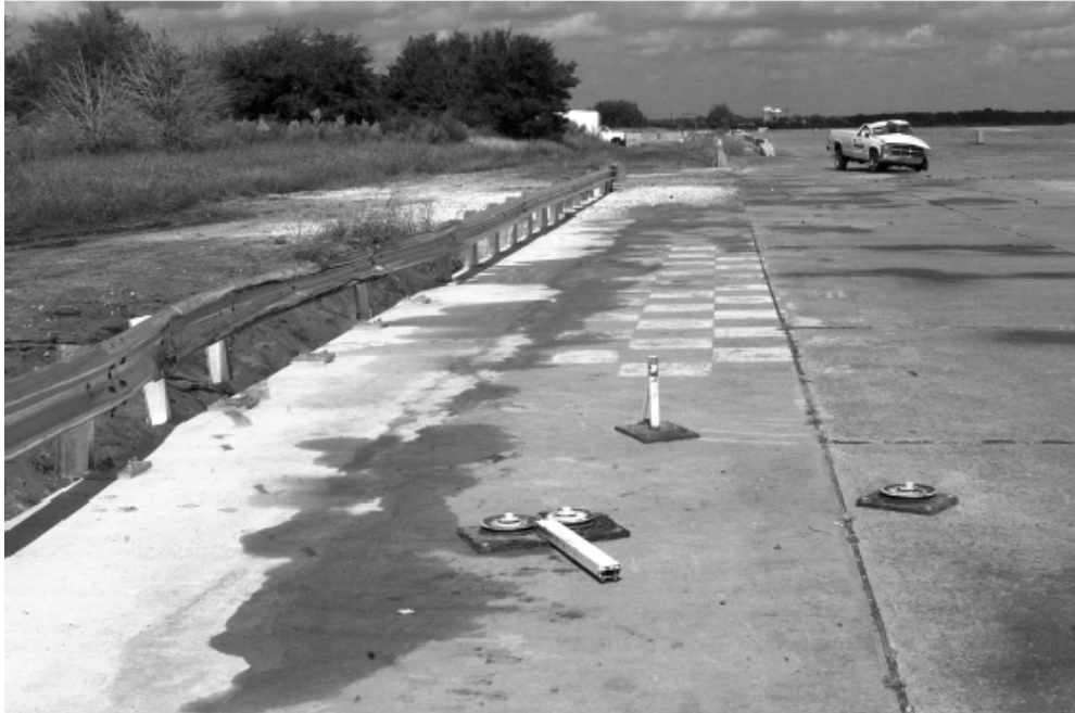
Figure 6. Rail Damage from Tubular W-beam Crash Test.
