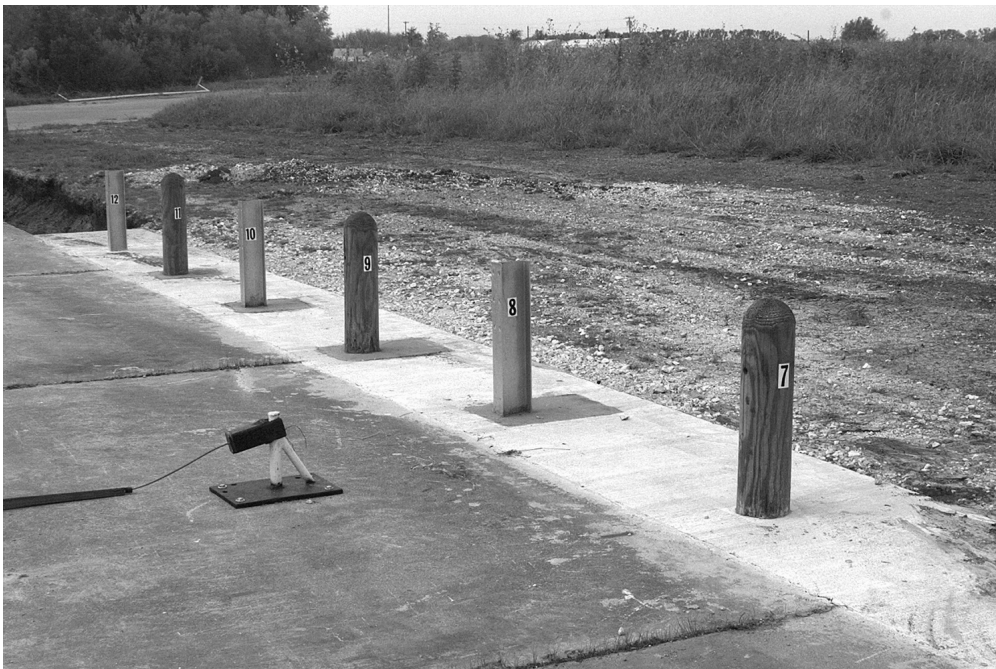
Figure 19. Concrete Mow Strip Installation Used for Dynamic Impact Tests.
