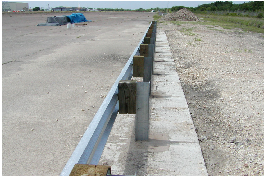
Figure 34. Completed Steel Post Guardrail Test Installation.
