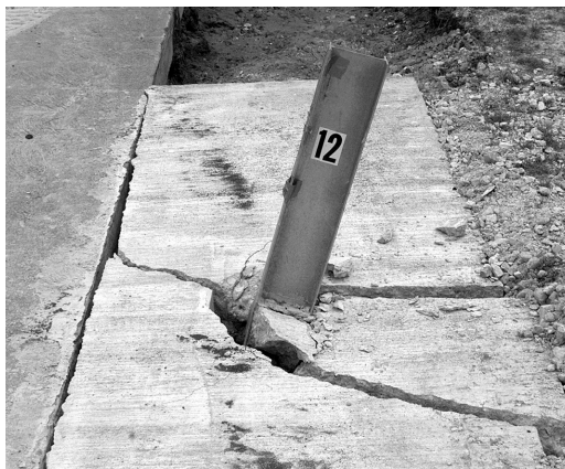
(a) Steel Post in Concrete
