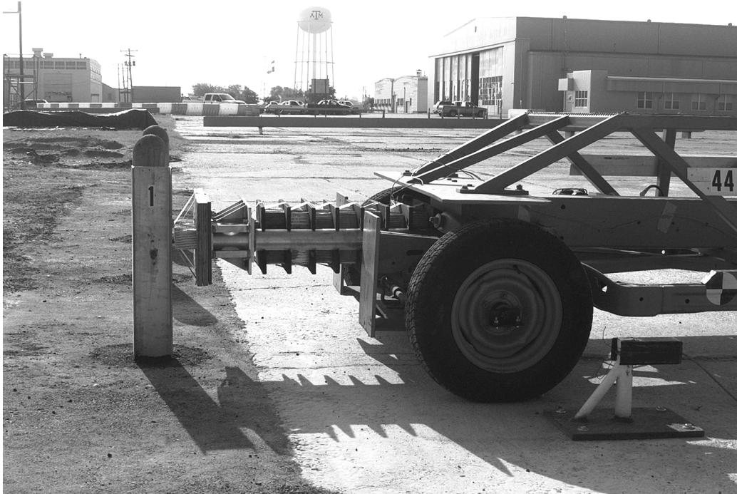
Figure 18. Asphalt Mow Strip Installation Used for Dynamic Impact Tests.
