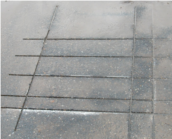
(c) Pavement after Saw Cut
