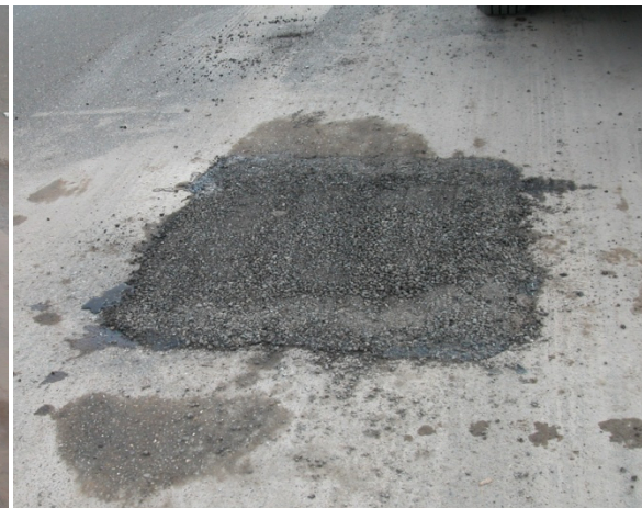
(f) Trench Filled up with Coldmix
