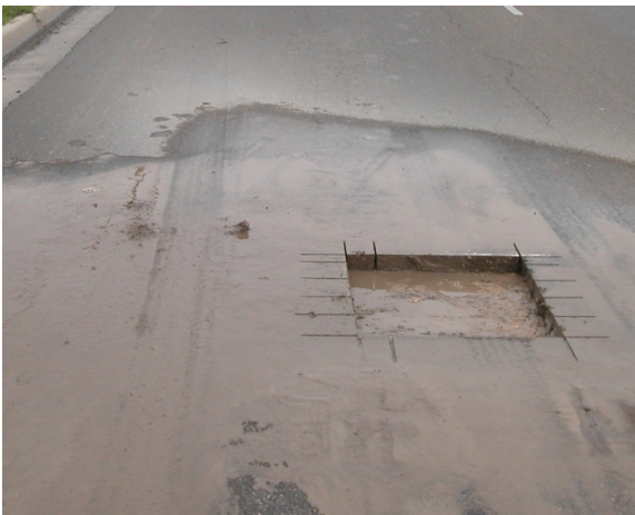
(e) Empty Trench
