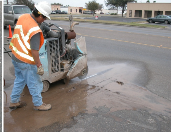
(b) Sawing Along the Template Marking
