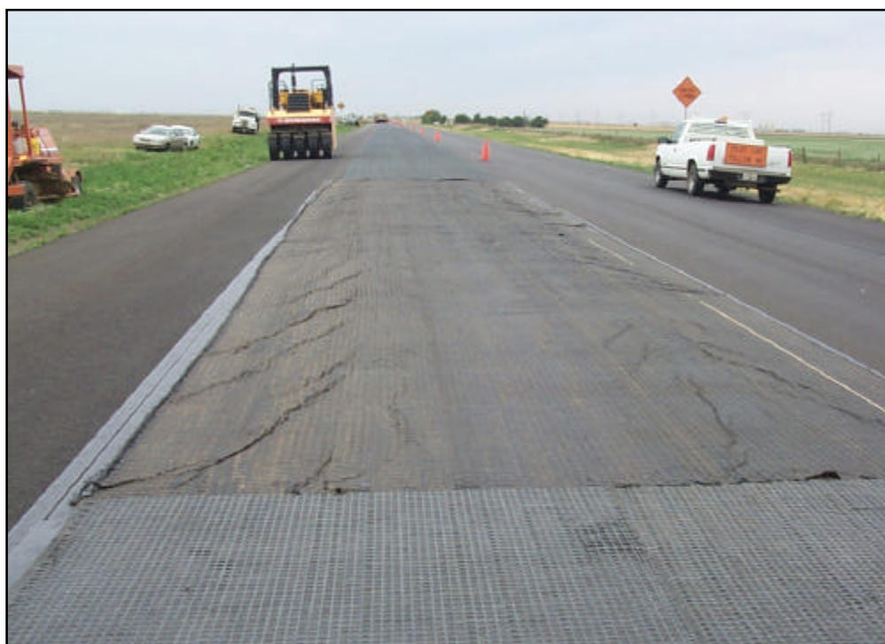
Figure 16. Wrinkles in 80-foot HaTelit Section.
