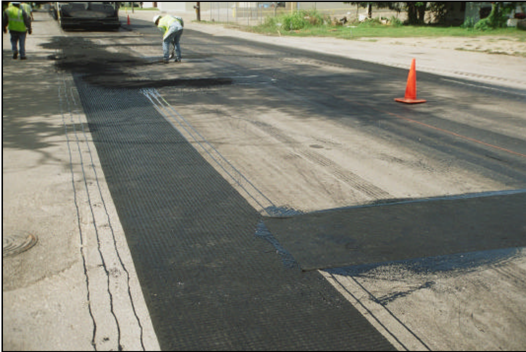
Figure 8. Marlin Project showing Geosynthetic Strips with No Tack between Them and Application of Loose HMA to Reduce Sticking to Construction Equipment Tires.
