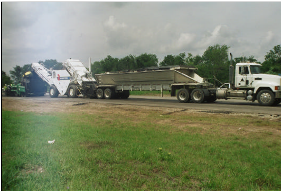
Figure 7. View of Paving Train at Bus 6 in Marlin, Texas.
