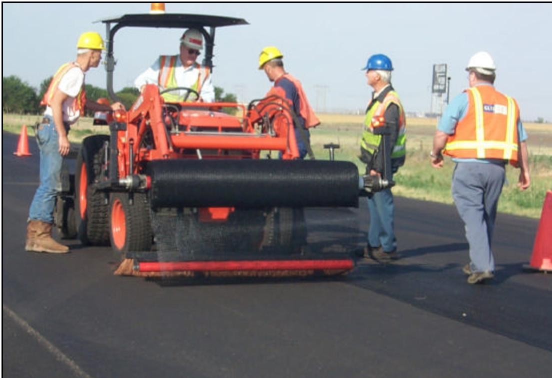
Figure 14. Placement of GlasGrid Product.
