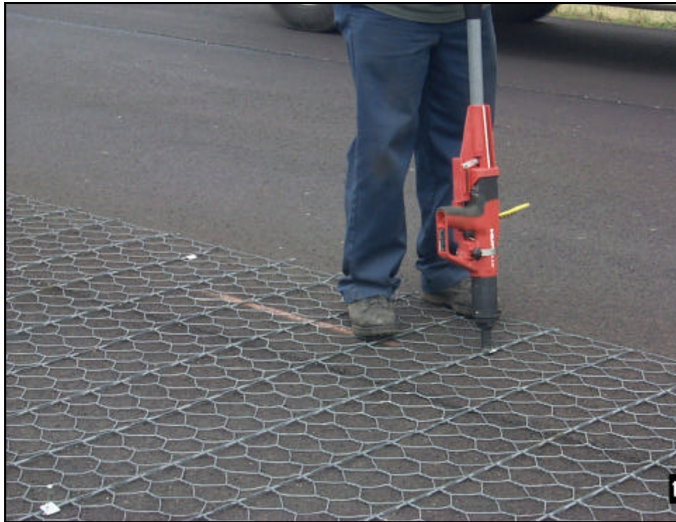
Figure 15. Anchoring Pavetrac Wire Mesh to Leveling Course Using Special Nail Gun.
