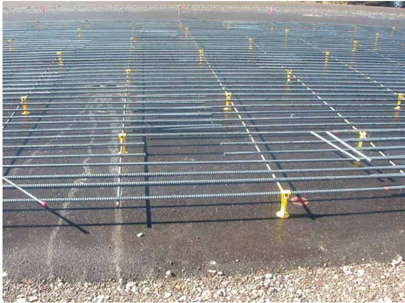
Figure A-2 Rebar Cutting for Instrumentation of Chilled Mirror Sensors.
