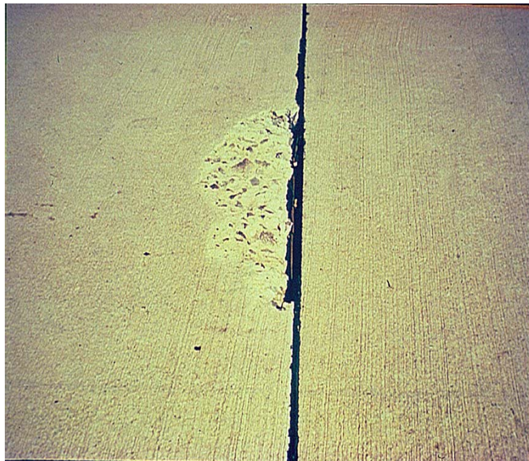
Figure 1-1 Spalled Joint.
