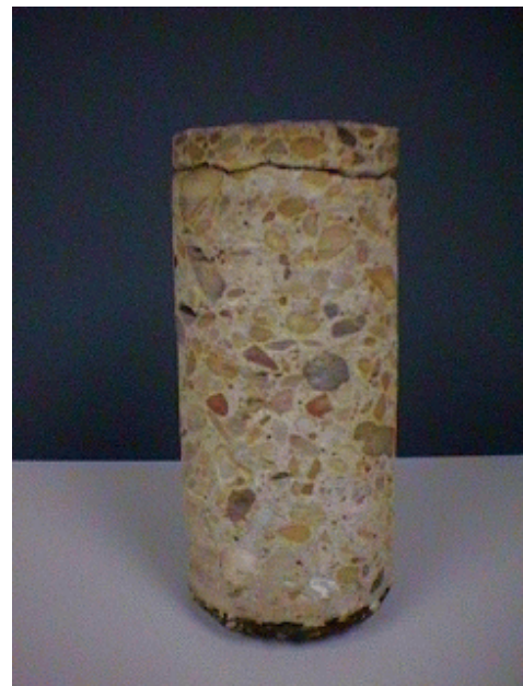
Figure 5-2 Delamination in an Unspalled Concrete Core.
