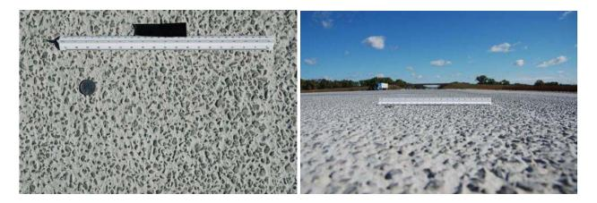
Figure 6. Exposed Aggregate Concrete (EAC) (Rasmussen 2008).
