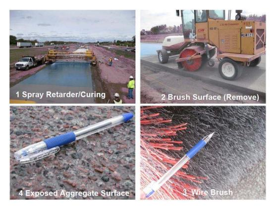
Figure 11. EAC Construction in Minnesota I-95 Project (Rao and Darter 2012).
