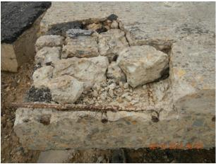
Figure 8. Two-Lift Pavement Delamination on I-30 at Sulphur Springs, TX (Photo Adopted from Dr. Moon Won).
