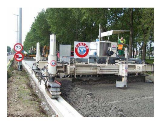
Figure 19. CRCP Construction in E34 Motorway Construction (Ren 2008).
