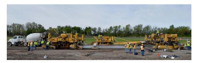
Figure 22. Paving Train Constructing R21 Research Sections along I-94 at MnRoad (Tompkins et al. 2011).
