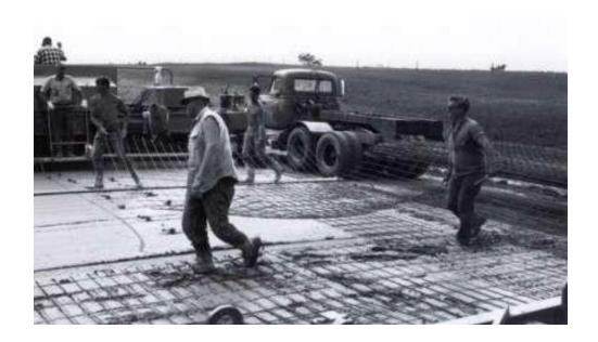
Figure 3. 2LCP with Welded Wire Mesh Reinforcement (I-80 Dallas County, Iowa 1966) (Grove and Taylor 2010).
