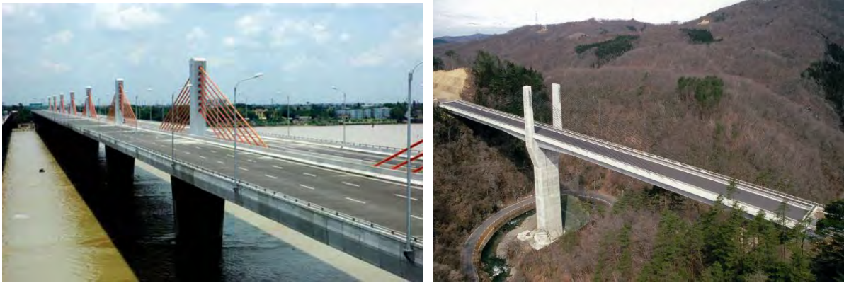
(a). Second Vivekananda Bridge (9 spans) (b). Yanagawa Bridge (2 spans)
