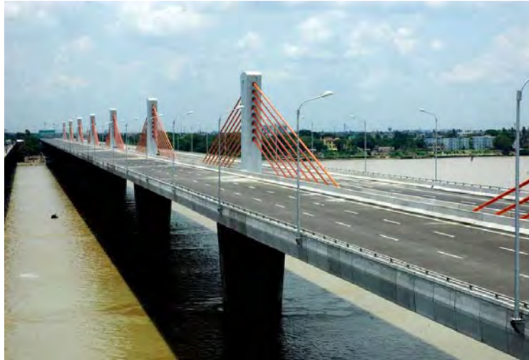
Figure 49. Example of Height Restriction to Fit Adjacent Structures (Second Vivekananda Bridge).
