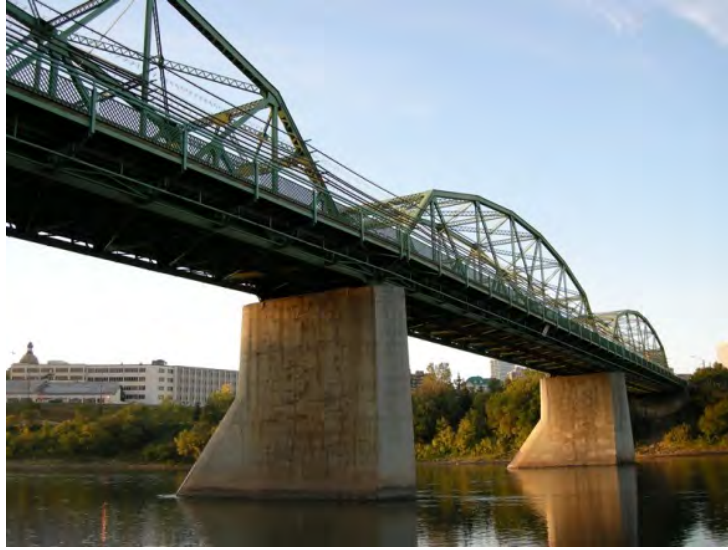
Figure 69. Existing Walterdale Bridge
