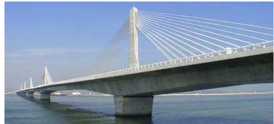
19 Ibi River (Ibigawa) Bridge (揖斐川橋) Japan 2001 (33) 505+891+891+891+891+515 98.4 (5x1) (14.1-24.0)x108.3 Hybrid cross section: four cell concrete box girder near piers and steel box girder in center with moment and shear connection
