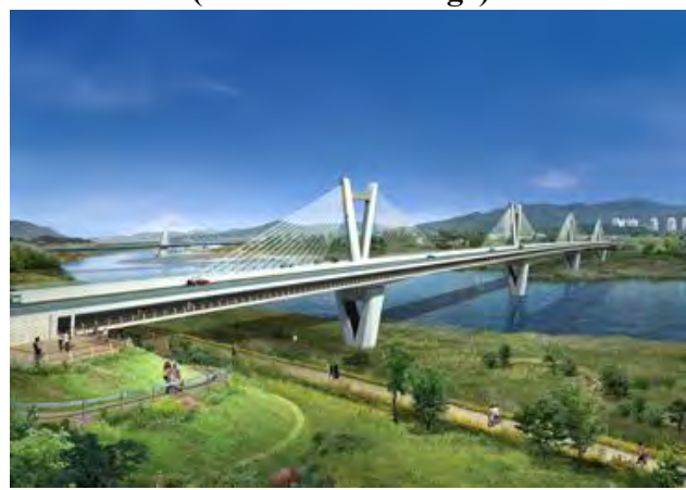
(d). Road and Pedestrian Hybrid (Guemgang I Bridge)
