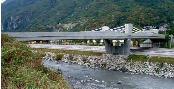
(a) Pont de Saint-Rémy-de-Maurienne Bridge (Main Span: 172 feet, Total Span: 311 feet)
