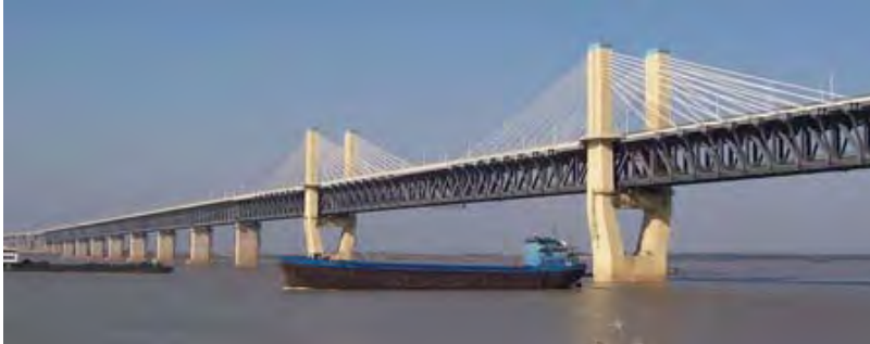
(b). Wuhu Yangtze River Bridge (with Constant Girder Thickness of 44.3 Feet)
