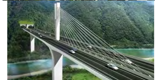
116 Naerincheon Bridge Korea 2015 394+509 -(1x1) -x100.1 Concrete box girder
