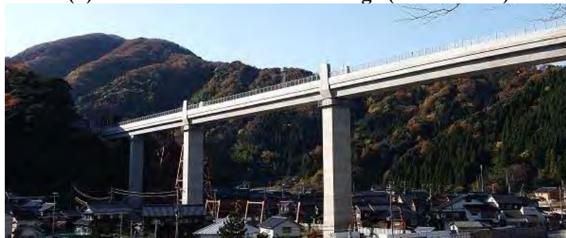
(b). New Amarube Bridge (Ratio of 16.5)
