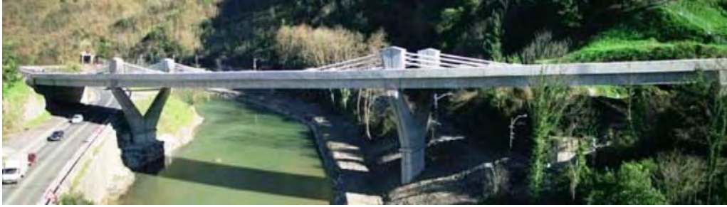
(a). Deba River Bridge (Constant Girder Thickness)
