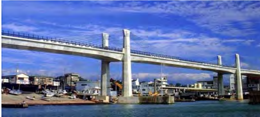
Figure 5. First Extradosed Bridge—Odawara Blueway Bridge.
