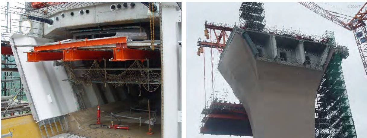
(a) Pylon and Pier Table
