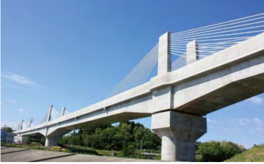
(a). Concrete girder–Sannai-Maruyama Bridge
