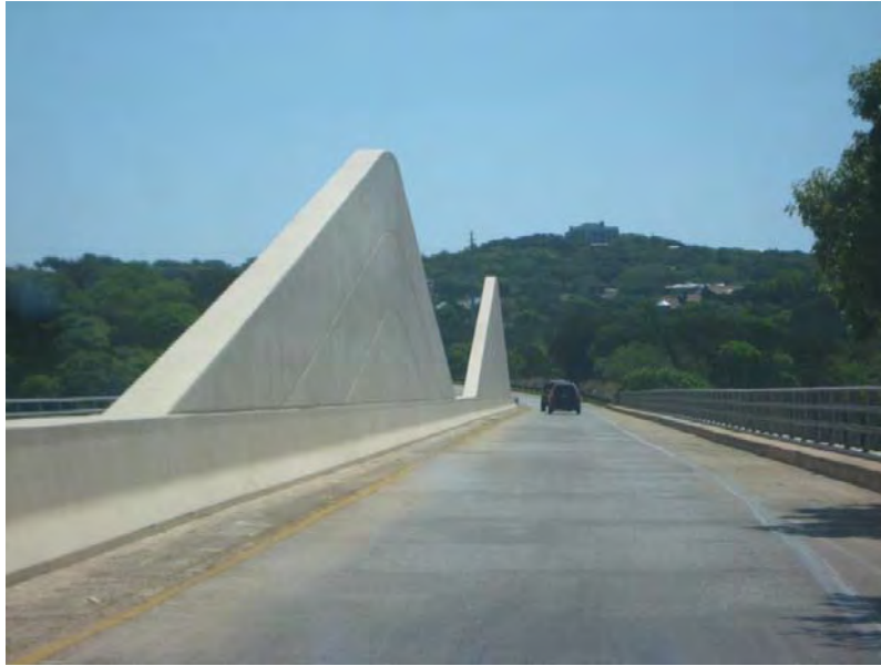
Figure 2. Finback Bridge–Barton Creek Bridge (photo from the Authors).
