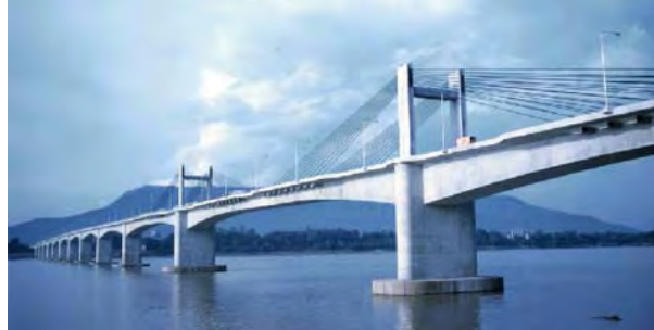
(b). Pakse Bridge (Variable Girder Thickness)
