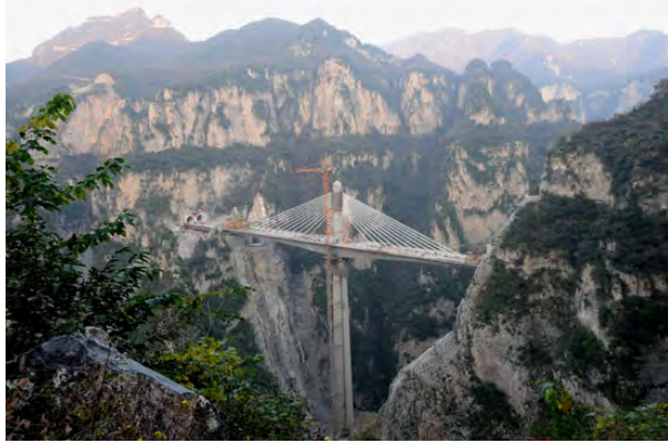
(a) Xianshen River Bridge (Tower Height 160.8 Feet)
