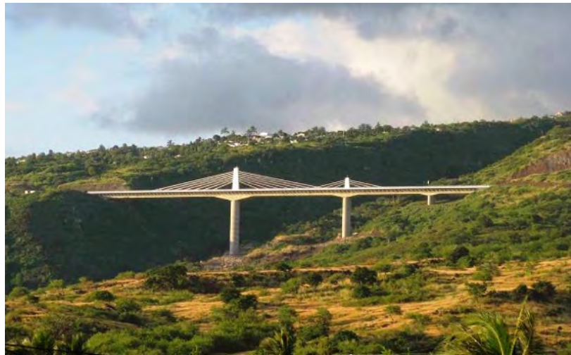
Figure 54. Example of Bridge with Span at Deep Valley (Trois-Bassins Viaduct).
