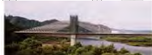
17 Yukizawa Bridge (雪沢大橋) 231+233 Japan 37.7 (2x2) 2000 (6.6-11.5)x51.8 Two cell concrete box girder
