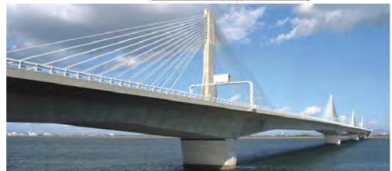
20 Kiso River (Kisogawa) Bridge (木曾川橋) Japan 2001 (33) 525+902+902+902+525 98.4 (4x1) (14.1-24.0)x108.3 Hybrid cross section: four cell concrete box girder near piers and steel box girder in center with moment and shear connection
