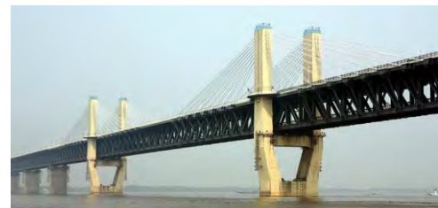
16 Wuhu Yangtze River Bridge (芜湖长江大桥) 591+1024+591 China 114.8 (2x2) 2002 (42) 44.3x76.8 Double-girderer steel truss with composite girder slab on top roadway, two rail lines on bottom level.
