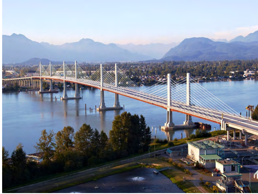
Figure 59. Example of Bridge with Structure Consideration (Golden Ears Bridge).
