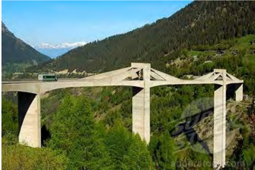
Figure 3. Cable-Panel Bridge–Ganter Bridge (photo adapted from lookbridges.com 2012).
