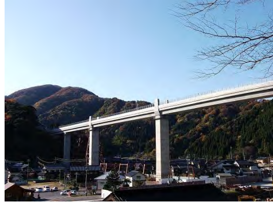
(b) New Amarube Bridge (Tower Height 16.5 Feet)
