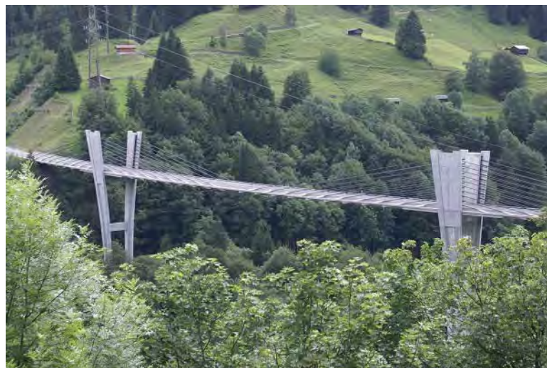
Figure 53. Example of Bridge with Low Visual Impact (Sunniberg Bridge).
