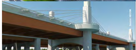
115 Brazos River Bridge United States 2015 185+185+185 46 (2x2x2) - x 56.5 (each direction) Continuous steel trapezoidal box girders
