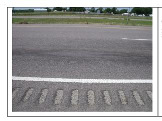
Cause is unknown but minor variation in the mix may have left a spot of softer binder allowing bleeding and raveling.
