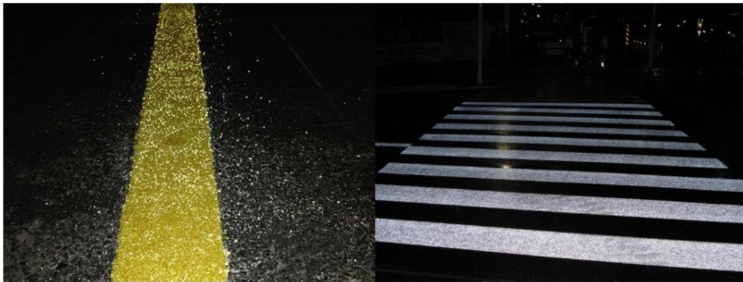
Figure 32 All-Weather Thermoplastic Retro-reflectivity During the Night (Source: Yeng Hsing Co., Ltd, 2020)
