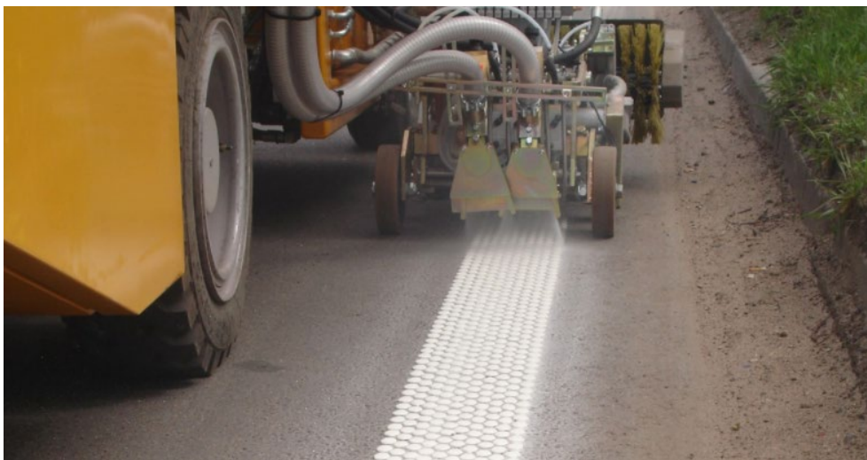
Figure 30 Dot Profile Marking Application Method
