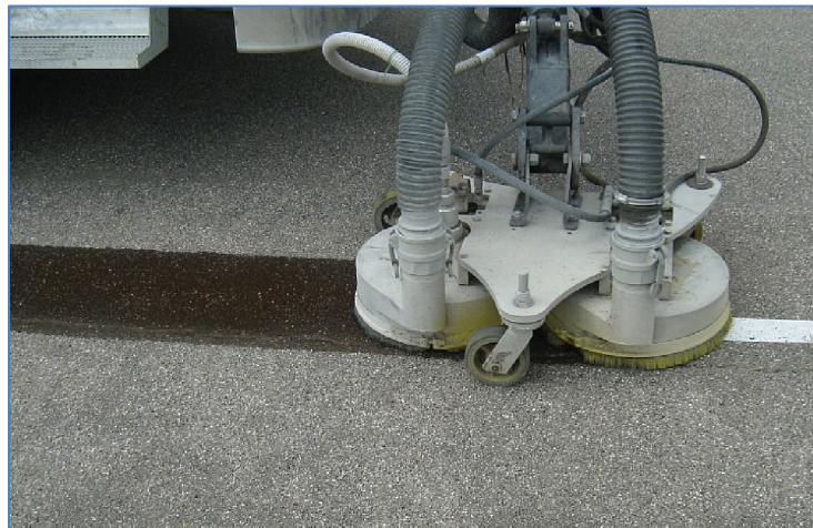
Figure 74 Water Blasting Paint Removal Equipment
