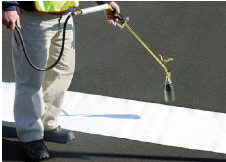
Figure 67 Arrow Symbol Being Applied by the Heat Torch (MnDOT, 2015)
