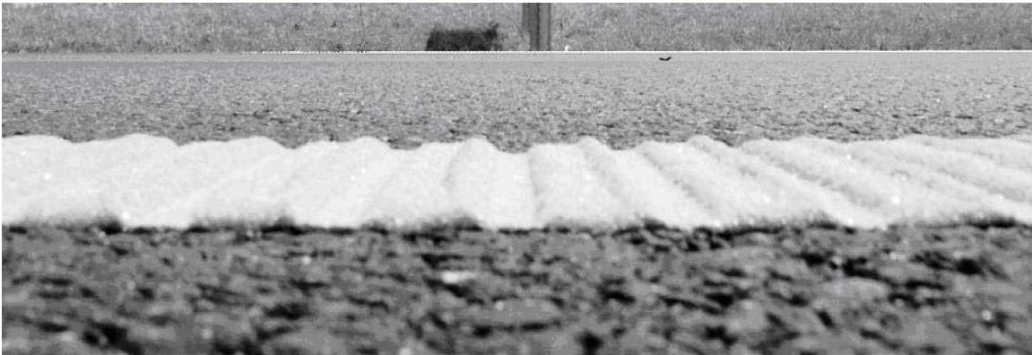
Figure 25 Typical Inverted Profile Thermoplastic Marking (Profile View)
