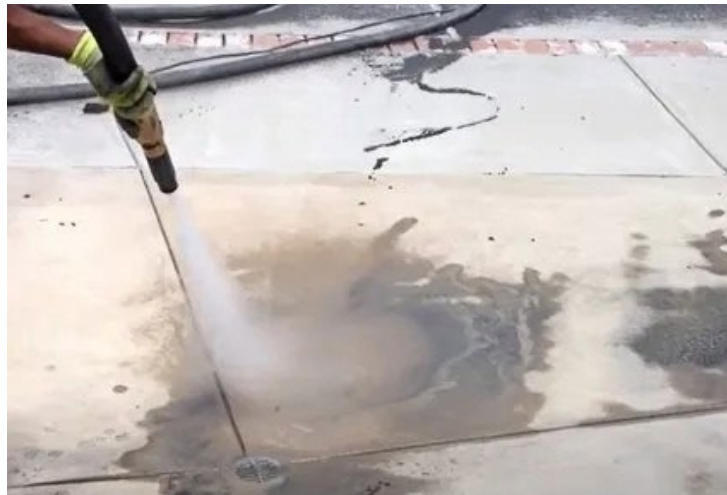
Figure 62 Sandblasting Equipment for Surface Preparation
