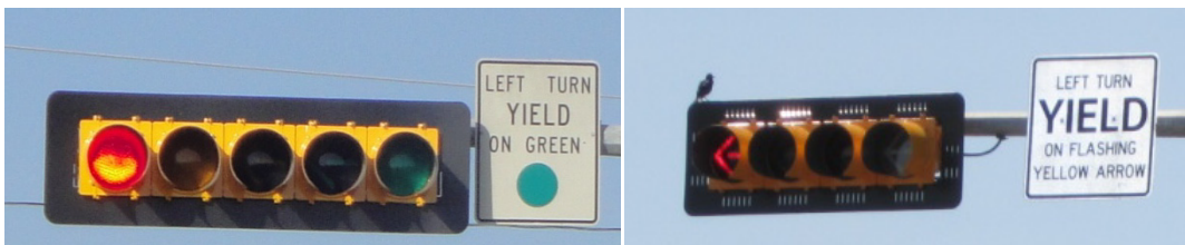
Figure 4-12: Before and After Arrangement of Left-Turn Signal Lens and Sign (Austin)
