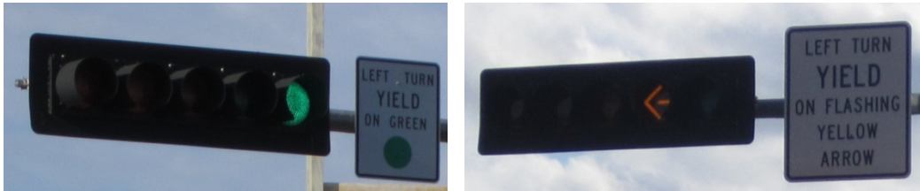
Figure 4-10: Before and After Arrangement of Left-Turn Signal Lens and Sign (Bellmead)
