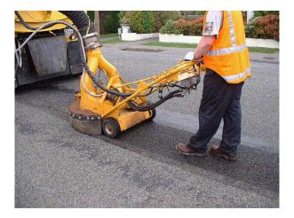
Though the water hits the pavement with enormous pressure, the machine uses a relatively low volume of water. The water removes excess asphalt and leaves the rock; the machine then vacuums up the water and the asphalt. After the process is finished, the watercutter is filled with about 95% asphalt and 5% water, which means that an insignificant amount of aggregate is pulled up.
