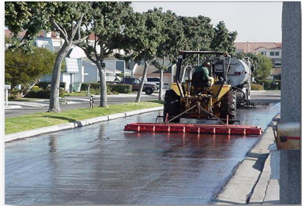
Residential Fog Seal Application
