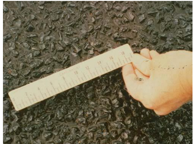
Fog Seal Atop Seal Coat Application
