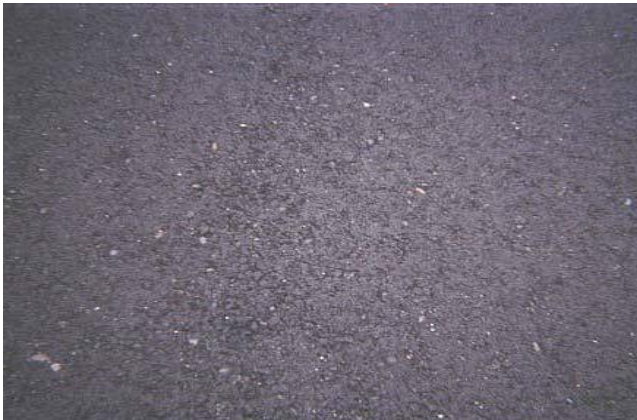
Dense Graded Surface - Not Suitable for Fog Sealing
