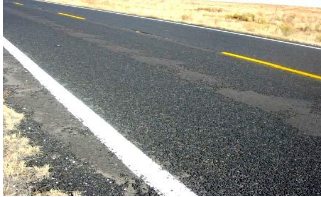
Seal Coat Four Years after Construction Left Lane = No Fog Seal Right Lane = With Fog Seal
