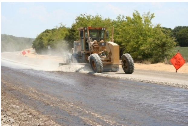
Figure 4- Worked-in (Cut-in) Prime
