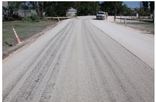
Figure 5- Covered (Inverted) Prime
