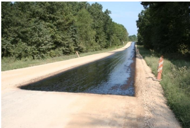
Figure 3- Spray Prime (MC-30, AE-P)
