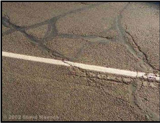
Figure 1: Crack Sealing
