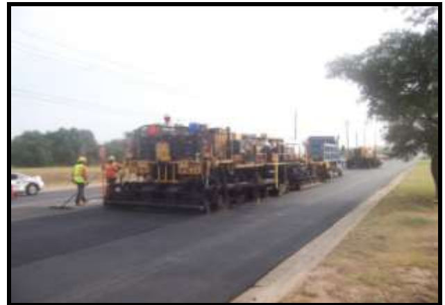
Figure 4: Hot-in-place Recycling
