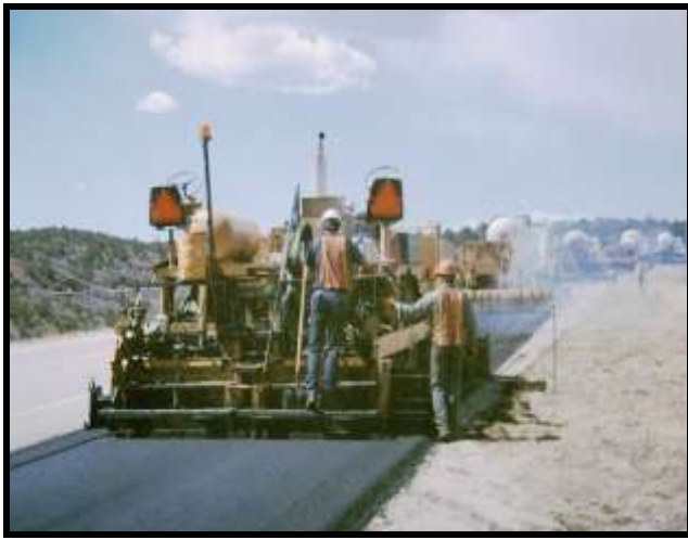
Figure 5: Thin asphalt overlay
