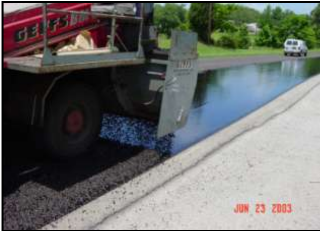
Figure 2: Seal coat application in progress
