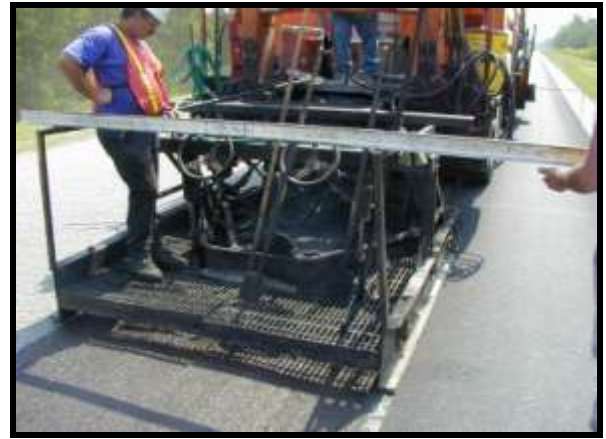
Figure 3: Micro-surfacing in progress
