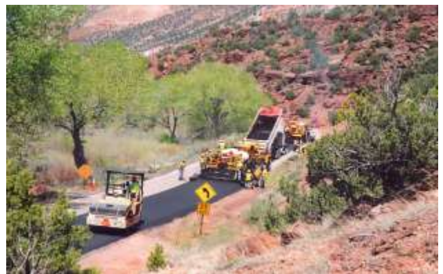
Mountain Pass Repaving Job
