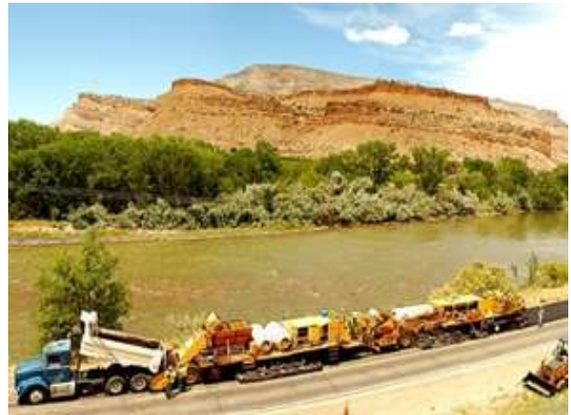
Cutler Once-Over Repaving Process
