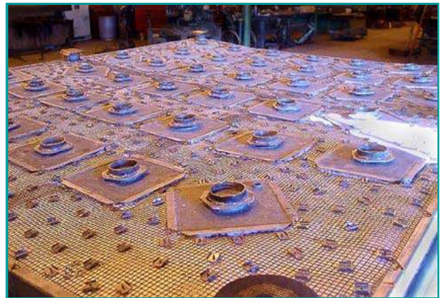
Underneath Heating Hood
