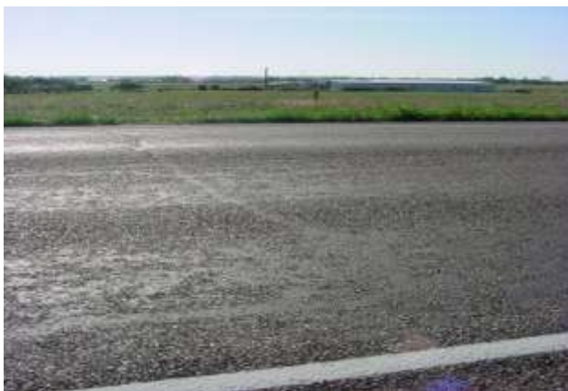
Test sections: Control section in background and section with Stress Absorbing Layer in the foreground
