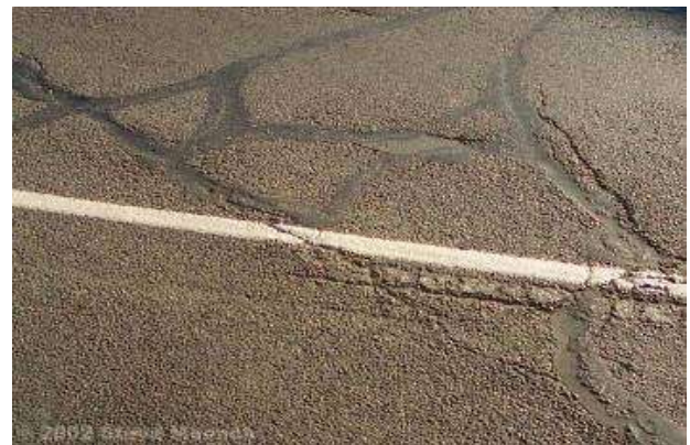
Pavement After Crack Sealing
