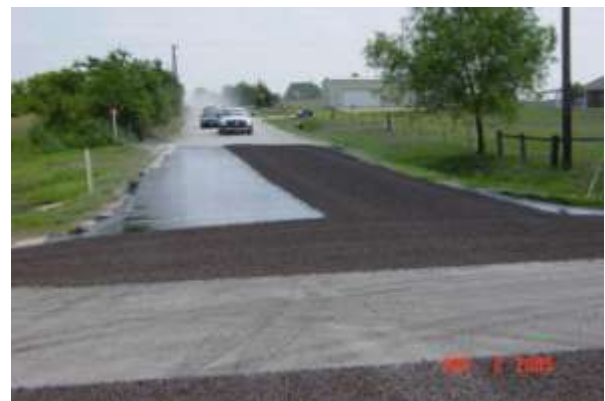
Chip seal job with tire rubber
