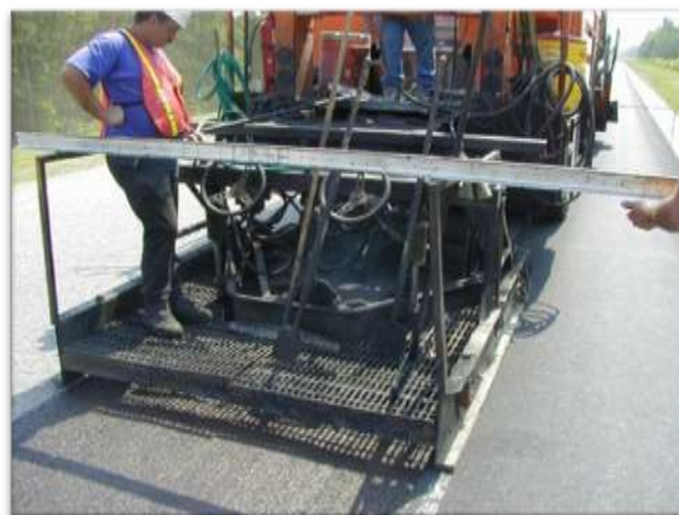
Microsurfacing and slurry seal
