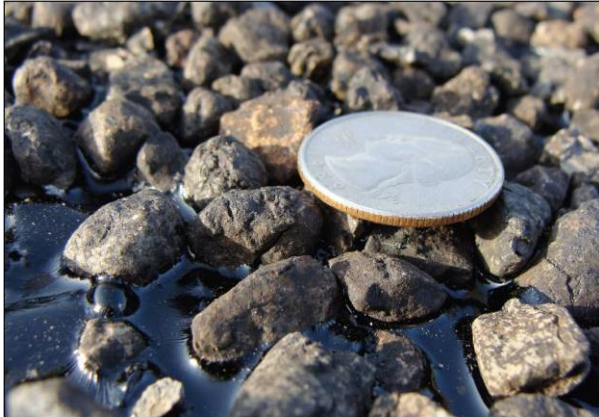
Figure 8. Embedment Slightly Higher than Desired
