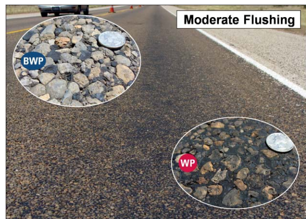
Figure 3. From the TxDOT Guide for TVAR, 2009
