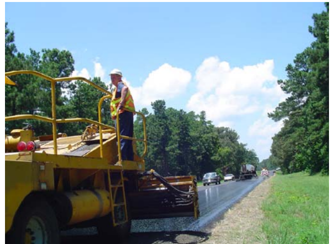
Seal Coat Application
