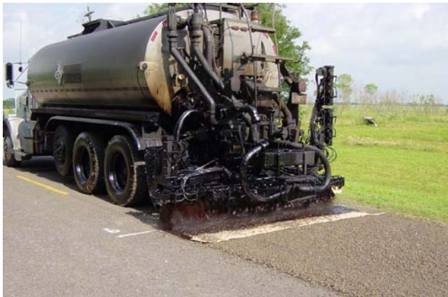
Seal Coat Application
