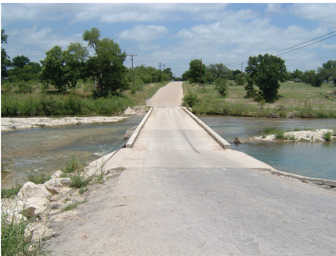
Figure 1. Flatrock Crossing of the South Llano River in Kimble County, Texas.
