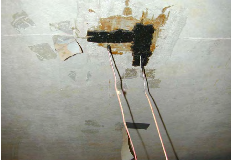
Figure 3.5 Surface Strain Gauges Centered on the Bottom of a Precast Concrete Panel
