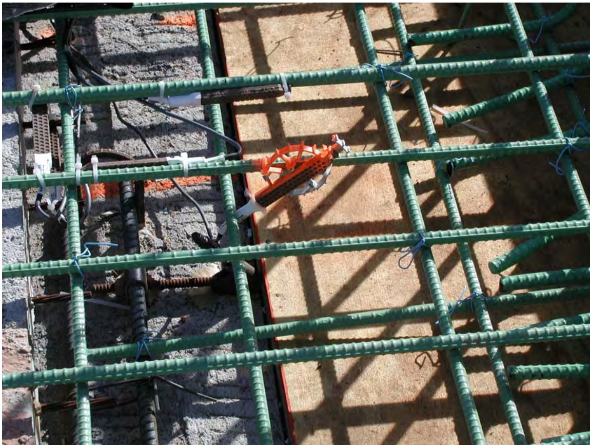
Figure 3.9 Embedded Strain Gauges at the Overhang of the Bridge Deck
