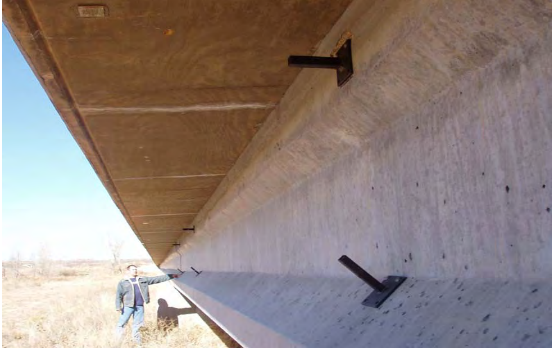
Figure D.1 LVDT Mounting Brackets on Span 6
