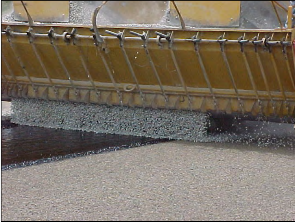
Figure 6.5 Application of Grade 3 Seal Coat Aggregate
