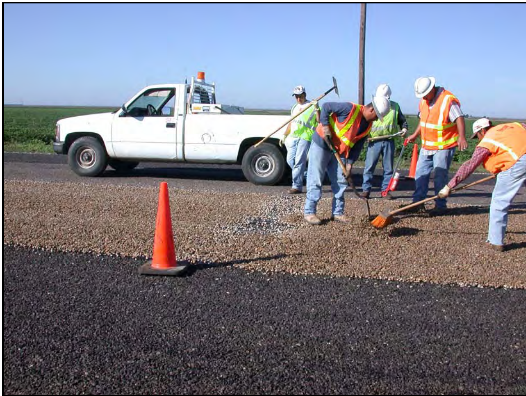
Figure 6.7 Hand Application of Aggregate to Treat Bleeding Pavement
