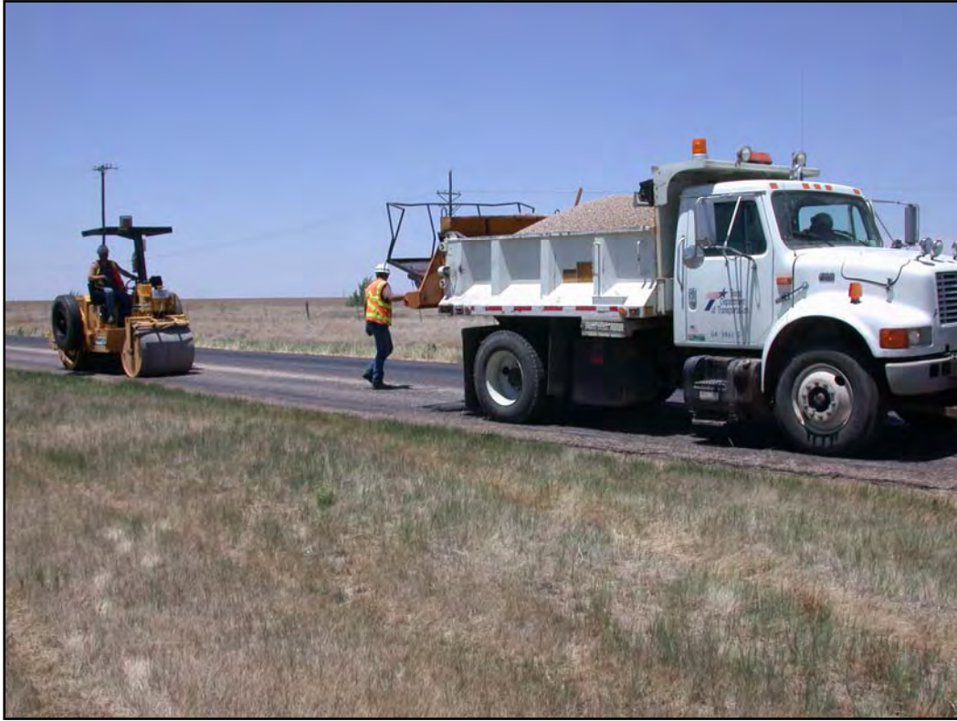
Figure 6.3 Application of Grade 5 Aggregate to Treat Bleeding
