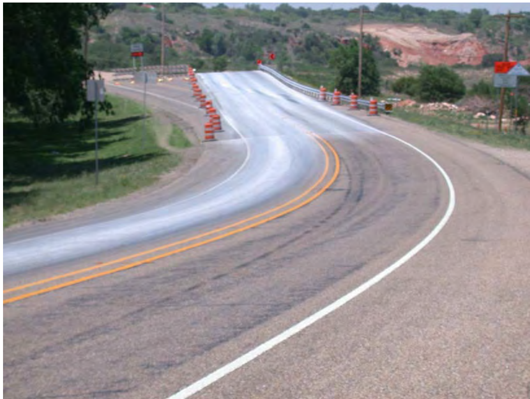
Figure 6.10 Application of Hydrated Lime to Cool Bleeding Pavement
