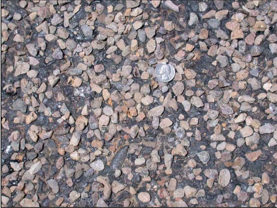
Figure 6.4 Grade 3 Aggregate to Treat Bleeding
