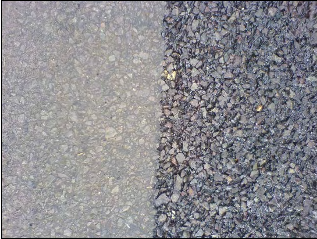
Figure 7.9 Ultra High Pressure Watercutting Allows Effective Removal of Excess Asphalt Binder Source: Fulton Hogan, Ltd. [ www.fh.co.nz ]
