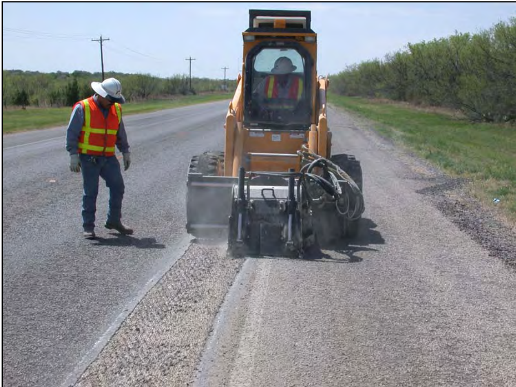
Figure 7.1 Cold Milling to Retexture Flushed Pavement in the Wheel Paths
