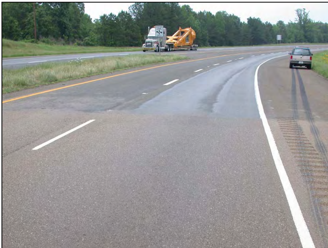
Figure 7.7 Thin Overlays to Treat Flushed Pavement Can Be Applied Using Asphalt Laydown Machines
