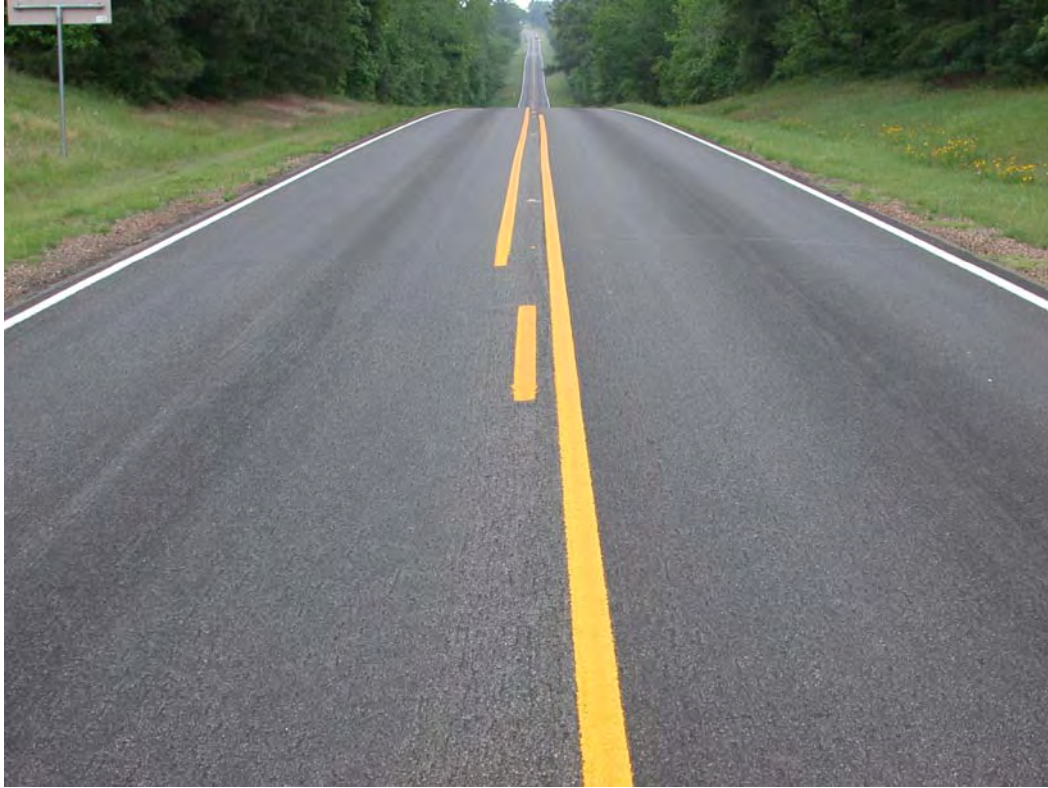
Figure 7.4 Microsurfacing Can Be Used to Remediate Minor Rutting, Flushed Pavement, Poor Ride Quality and Low Skid Resistance
