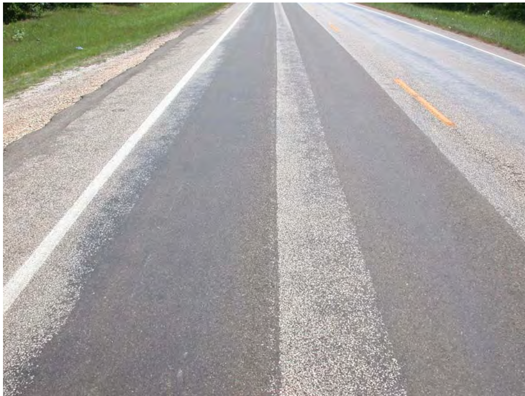
Figure 6.8 Sandwich Seal Used to Treat Bleeding Pavement in the Wheel Paths
