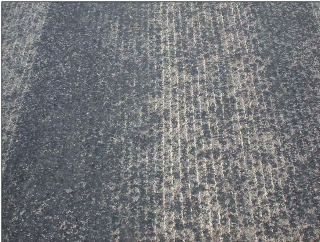
Figure 7.10 Grooves in a Motor Grader Mold Board Can Score the Flushed Pavement to Improve Surface Texture
