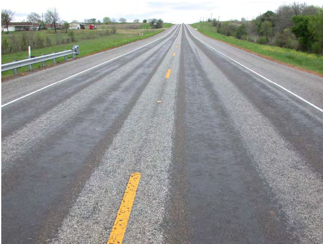
Figure 7.3 Strip Seals (a New Seal Coat in Wheel Paths) to Control Flushed Pavement Must Be Carefully Designed to Avoid Additional Flushing
