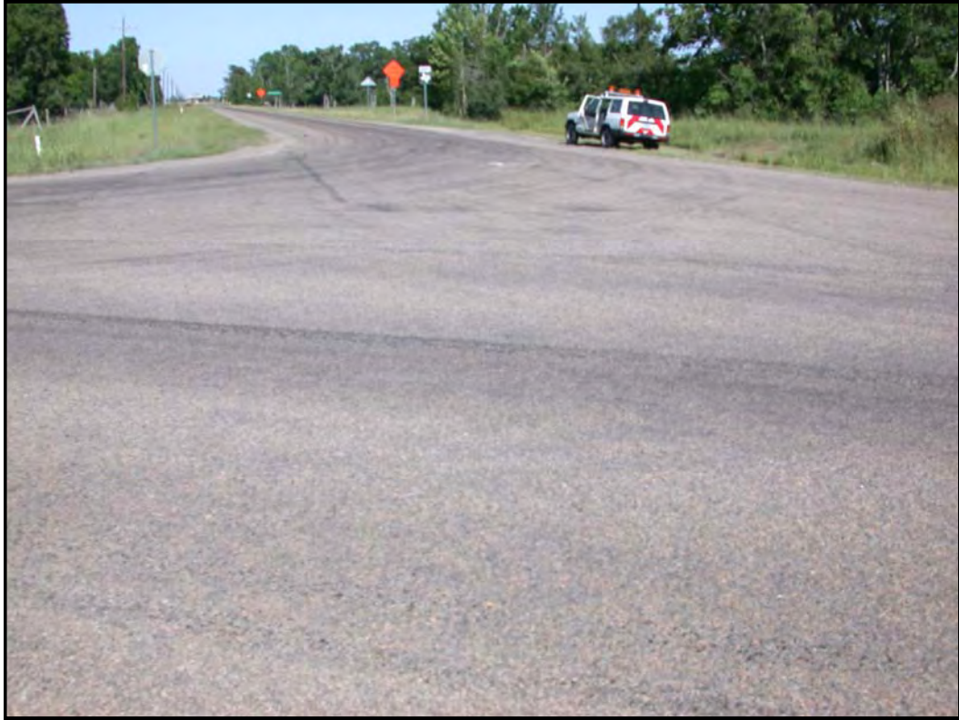
Figure 8.2 The Racked-In Seal Can be Used at Intersections to Improve Seal Coat Performance Under Heavy Traffic or Abusive Traffic
