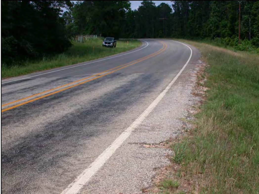
Figure 7.6 Blade Level-ups and Other Thin Asphaltic Concrete Overlays Restore Friction and Skid Resistance
