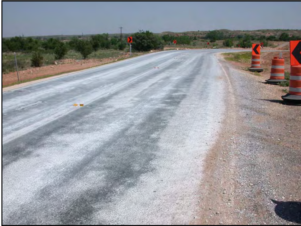
Figure 6.13 Lime Can Obscure the Reflectability of Pavement Markings and Striping
