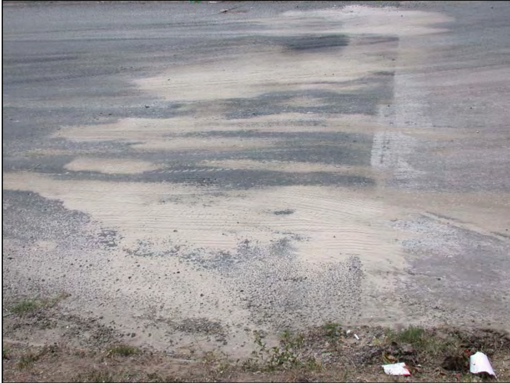
Figure 6.6 Application of Sand Blotter Material to Treat Bleeding Pavement at an Intersection
