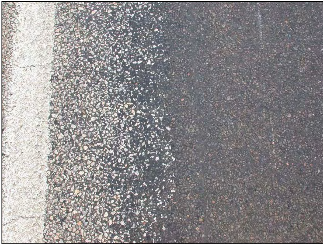
Figure 6.9 Improved Macrotexture in the Wheel Paths Using a Sandwich Seal
