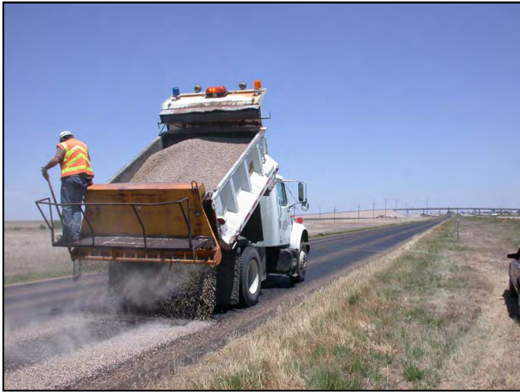
Figure 6.1 Applying Small-Size Aggregate to Treat Bleeding Pavement
