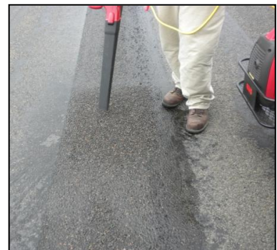
(c) drying of treated surface prior to CTM testing
