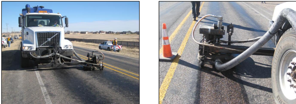
FIGURE 1.1 UHP water cutter with a fixed cutting head attachment
