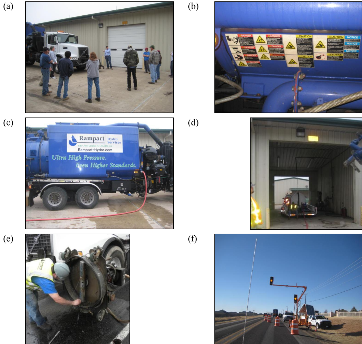
FIGURE 2.6. Daily operations for Ultra High Pressure (UHP) Water Cutter treatment (a) safety meeting at TxDOT maintenance yard; (b) hazard warnings in the water cutter truck; (c) pumping water into the water cutter truck; (d) getting water to the 4000-gallon water cutter truck - using water trailer when there is insufficient overhead clearance for the truck; (e) adjustment of water cutter spray bar and nozzles prior to treatment; (f) traffic control for the treatment operation by closing the treatment lane.
