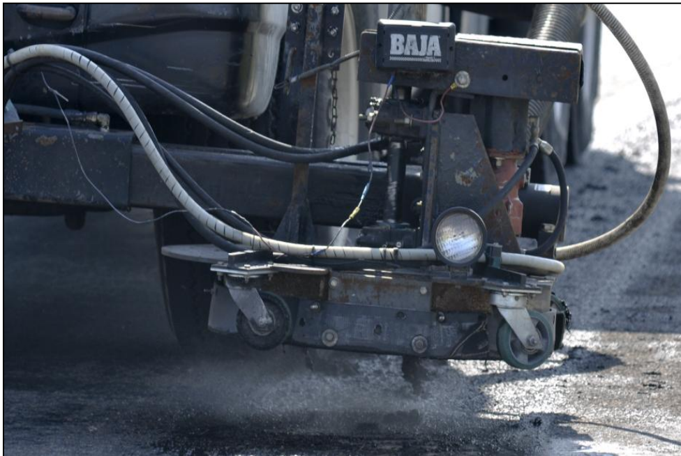
FIGURE 4.4. Cutting head, Rampart BlasterVac. Image courtesy Chris Sasser, TTI Visual Media.
