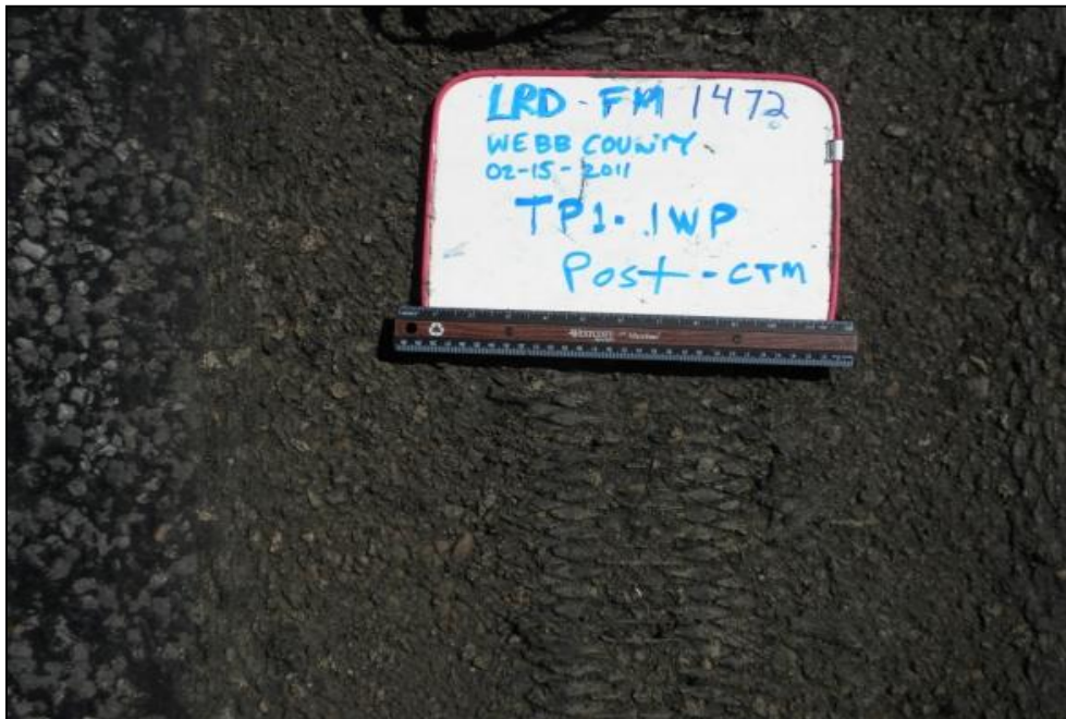
FIGURE 4.9. "Holiday" areas not subjected to treatment due to ineffective nozzle coverage, in this case along the center of the treatment path
