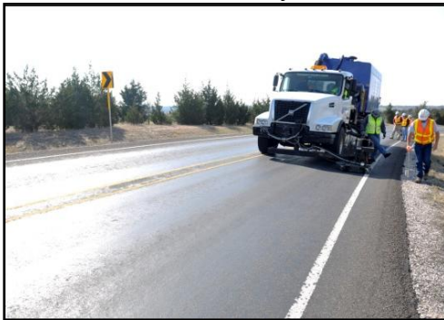
(c) Initial pass, UHP water cutter
