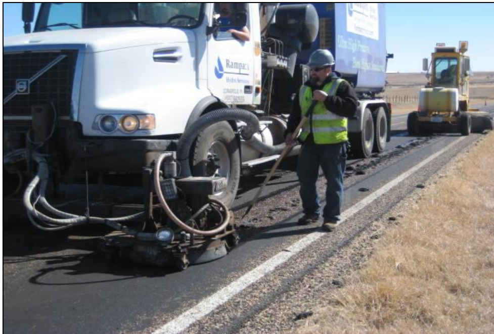
FIGURE 4.10. Maintenance worker using a shovel to remove excess lumps of asphalt
