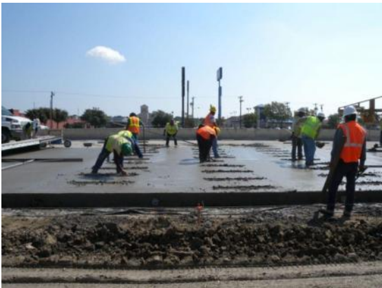
Figure 2.8 Removing concrete from the top of stressing pocket cover
