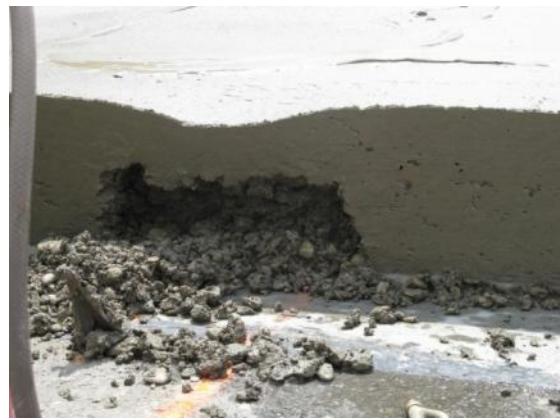
Figure 2.9 Edge slump due to the removal of concrete for the space for the connection of transverse bars
