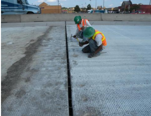
Figure 2.11 Chipping concrete to expose grouting hoses at armor joints
