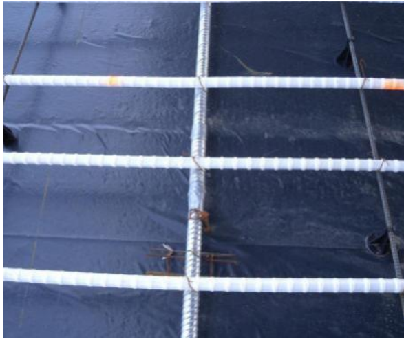
Figure 2.6 Bar installed to keep transverse post-tensioning bar in place
