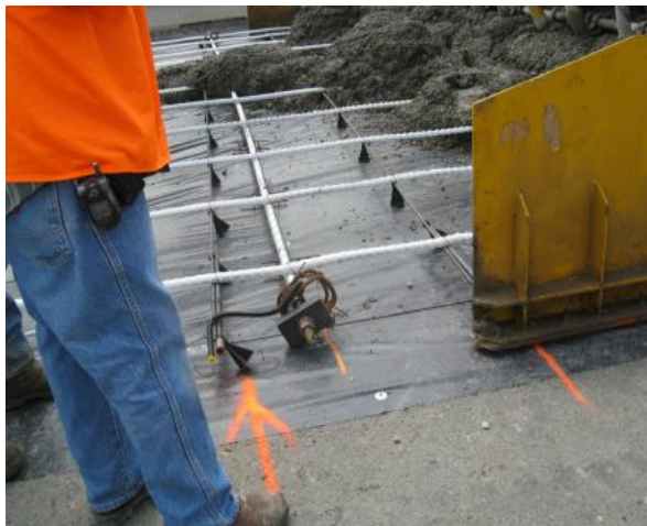
Figure 2.2 Tendons and transverse bars pushed by concrete
