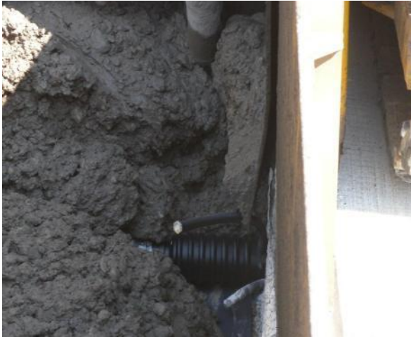
Figure 2.10 Grouting hose at longitudinal construction joint not interfering with placement
