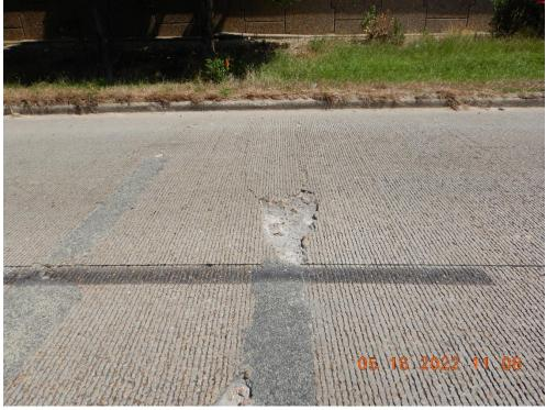
Figure 2.1 Typical spalling in CRCP observed in Texas
