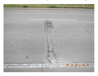
Figure 3.4 Distress caused by horizontal cracking on IH 35
