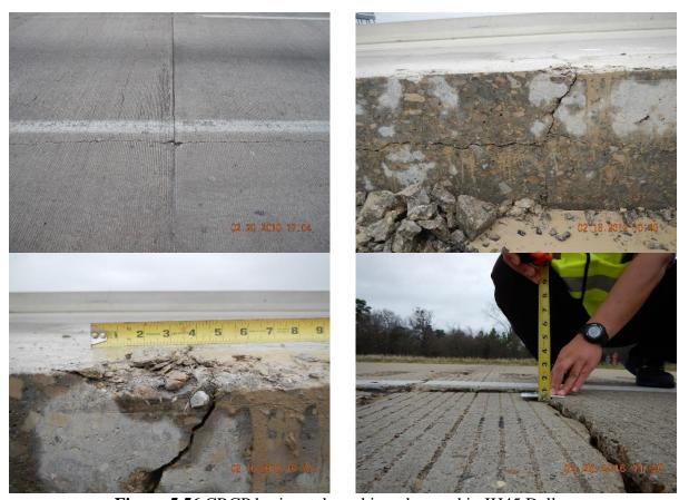
Figure 5.56 CRCP horizontal cracking observed in IH45 Dallas
