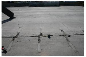
Figure 5.51 CRCP expansion and resulting stapling failure
