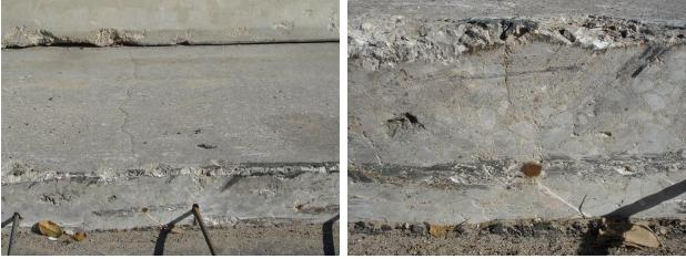
**Figure 2.15**-(a) Wide crack width on the slab surface (left); (b) Transverse crack profile through slab depth (right)
