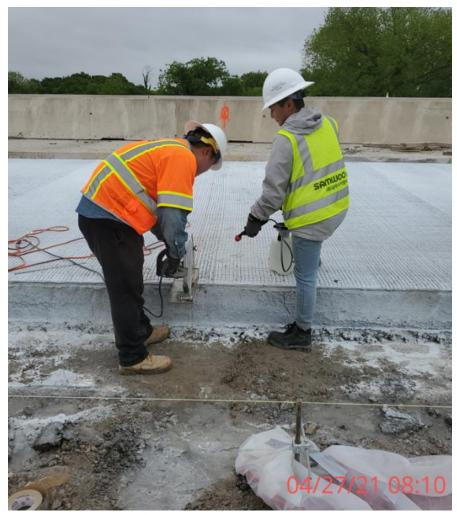
Figure 5.19 Sawcut operation
