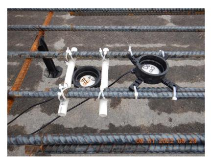
Figure 5.6 REBEL Sensor and its typical installation
