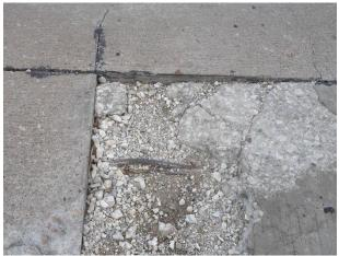
**Figure 2.11**-(a) Stapling failure due to slab expansion (left); (b) Failure of full-depth repair due to slab expansion (right)
