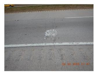
Figure 3.3 Distress caused by horizontal cracking on IH 20
