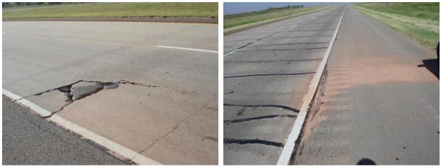
**Figure 2.7**-(a) Punchout distress on US 287 in Harrold (left); (b) Severe pumping on US 287 in Harrold (right)
