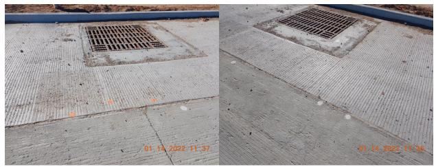
Figure 5.91 Development of reflection cracking at SC #1 from the drainage manhole
