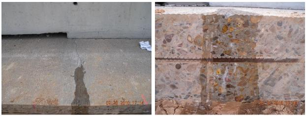
**Figure 2.14**-(a) Wide crack width on the slab surface (left); (b) Transverse crack profile through slab depth (right)
