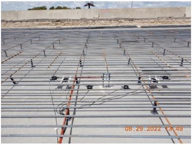
Figure 5.16 Actual gauge installation location at STA 212+00 in Hillsboro
