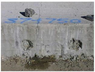
Figure 3.1 Horizontal cracking in new CRCP
