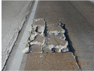
Figure 2.8-(a) Punchout distress on Loop 610 (left); (b) Punchout on Loop 610 (right)
