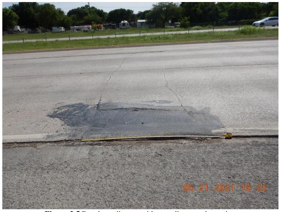
Figure 2.5 Punchout distress with a medium crack spacing
