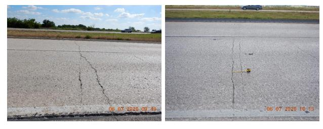
Figure 2.4-(a) Y-crack with no distress (left); (b) Short crack spacing (right)
