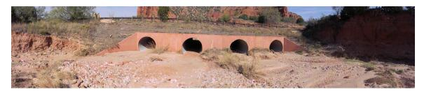
Figure 1: 4-Barrel Culvert System at Caprock Canyons State Park (G.R. Herrmann)
