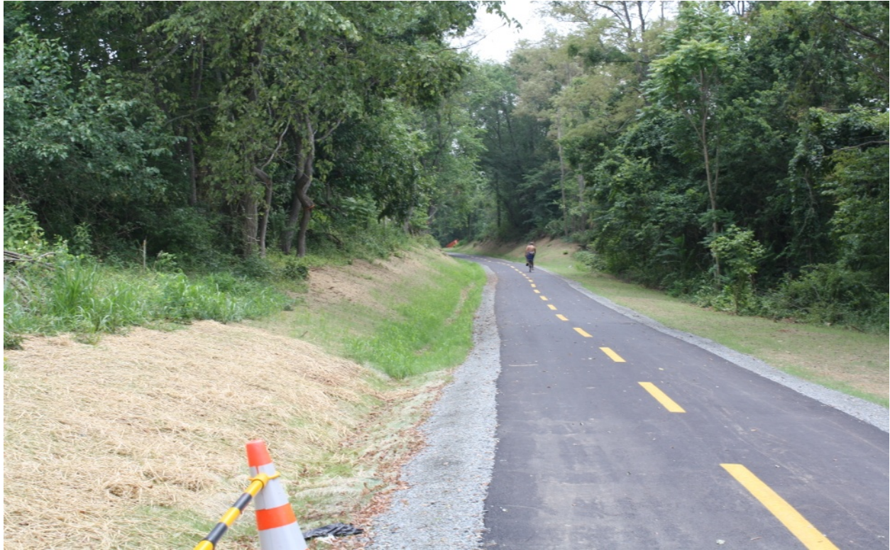
Figure 4.6 Mitigation - Detour Bike Trail Paved by Dominion
