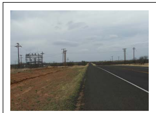
Figure 1.2 2183 kV transmission line, sub-station and 12.5 kV distribution line crossing a state highway
