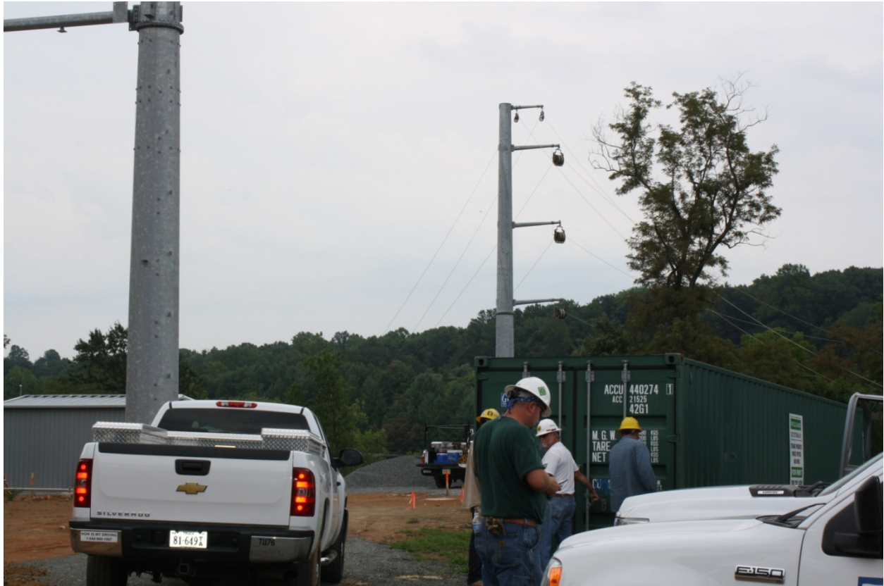
Figure 4.7 Hamilton Substation Construction Site
