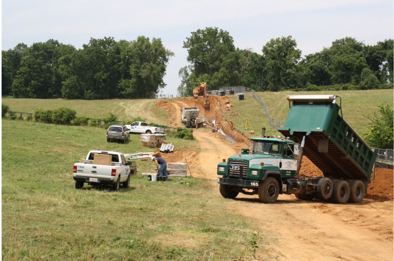
Figure 4.5 Laying of Underground HV Cable
